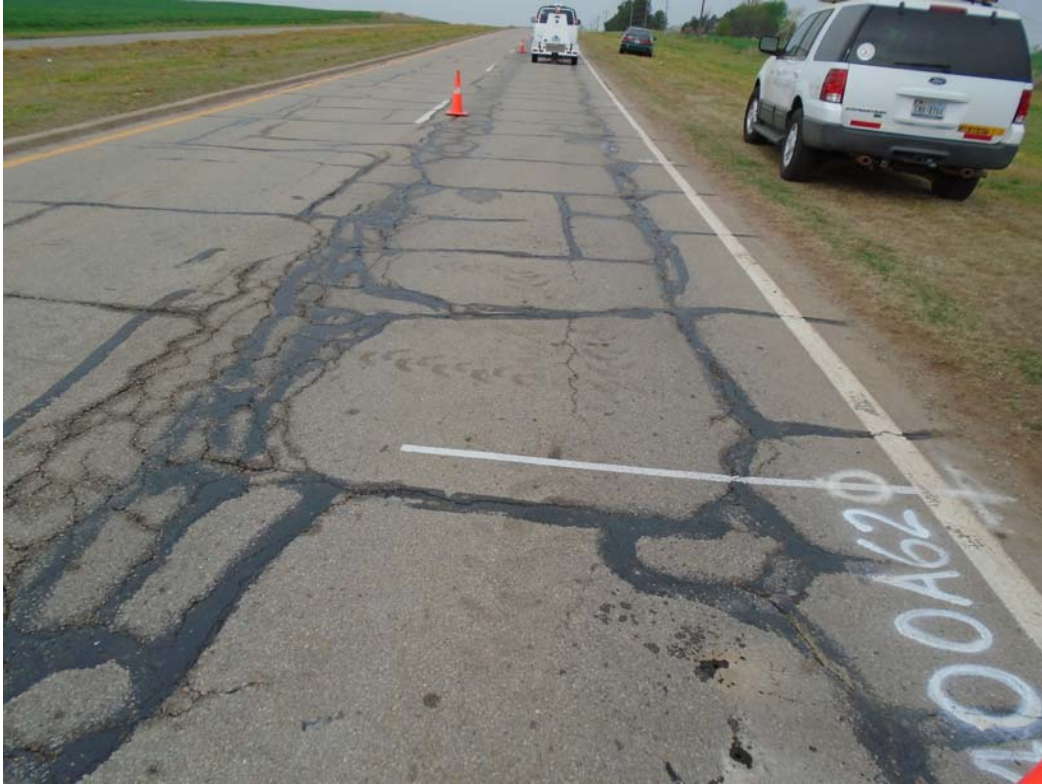
Figure 8. Image of section 40_AA62 in April 2015 at station 0+00 prior to overlay showing severe level of cracking. This test section was rated as having block cracking and no transverse cracking.
