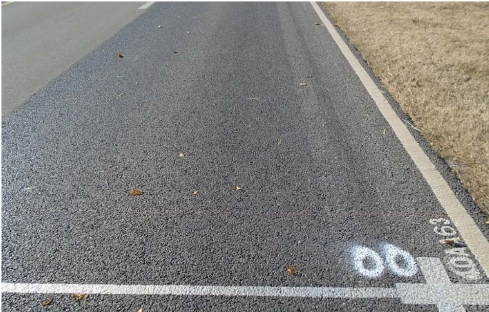
Figure 11. Image of section 40_AA63 in 2016 showing the new as-placed SMA mixture in the right lane. Note the tight center-lane longitudinal joint and different surface type uses in the left lane.
