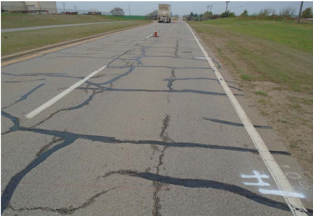
Figure 15. Preoverlay image of section 40_AA61. This section has a similar cracking pattern to section 40_AA62, shown in figure 8 that were rated as block cracking. The transverse cracks on this test section were rated as transverse cracks.
