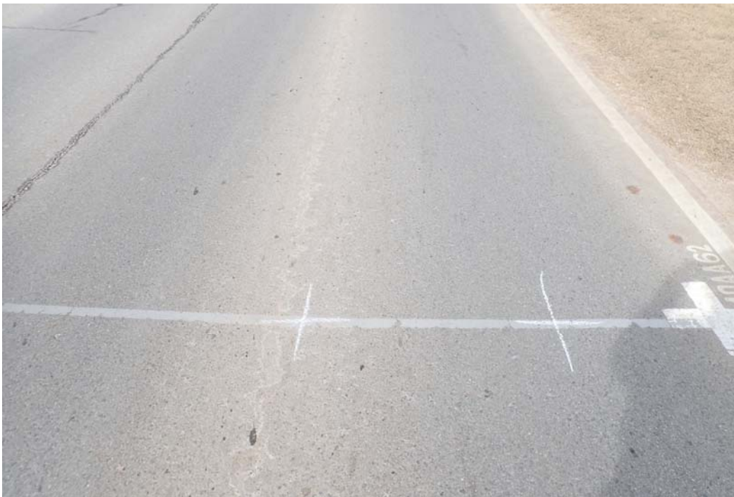
Figure 9. Image of test section 40_AA62 in March 2019 at station 0+00 approximately 3.5 years after mill and overlay. The longitudinal chalk lines show lane center and middle of right wheel path, where the line of FWD measurements will be performed along the test section.
