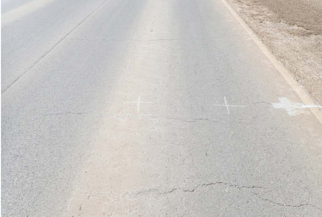
Figure 16. Image of Section 40_AA62 in March 2019. This is an image of the same portion of test section as shown in figure 15. The location and pattern of the cracks support the reflection cracking hypothesis. This test section had the highest amount of post-overlay transverse cracking in 2019.
