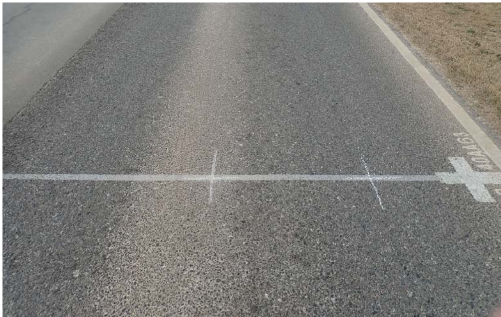
Figure 12. Image of section 40_AA63 in 2019, when the between lane longitudinal joint is now rated as a full test section length NWP longitudinal crack.
