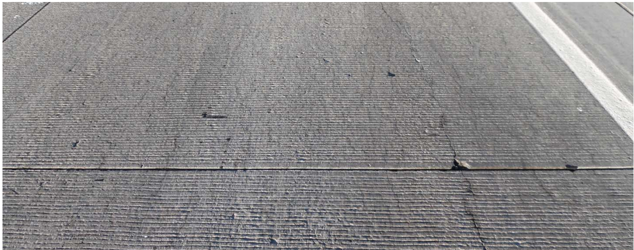
Figure 17. December 2015 image of joint on test section 20_0206 at stations 26 feet (8 m). Image shows potential masking of short longitudinal cracking over dowel bars rated as map cracking.
