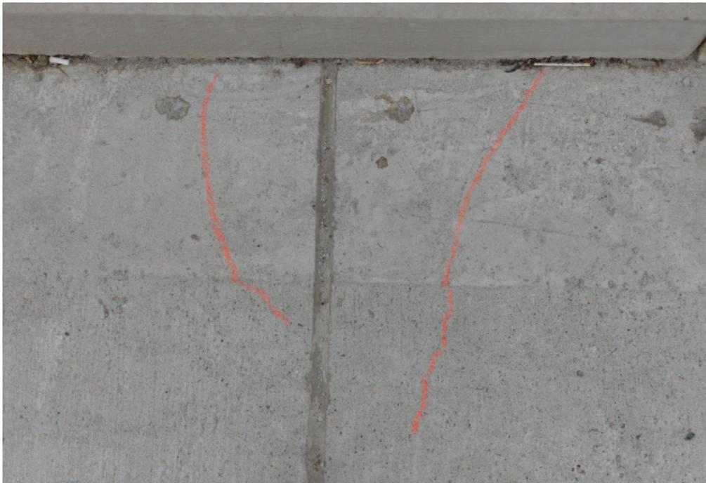
**Figure 3.1: IC-LC-HPC-1 Typical Crack Pattern**
