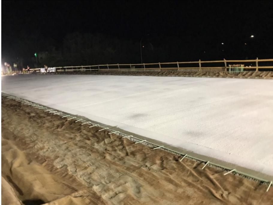
**Figure 2.10: Finished IC-LC-HPC-4 Deck Showing Spots of Uneven Curing Compound Application**
