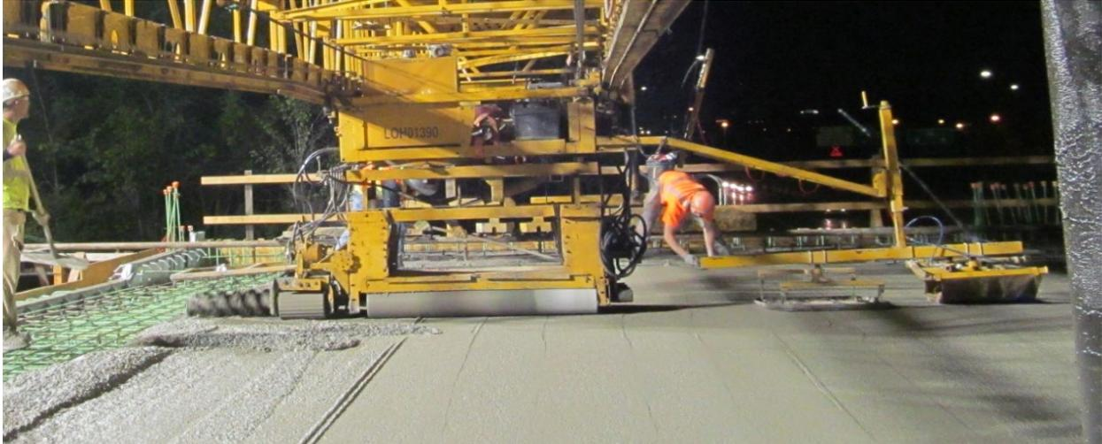
**Figure 2.8: IC-LC-HPC-4 Finishing Equipment**
