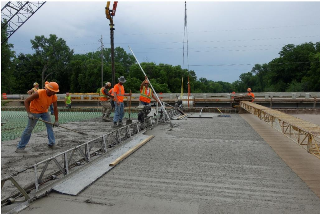
**Figure 2.4: Placement, Finishing, and Curing Setup for IC-LC-HPC-2**
