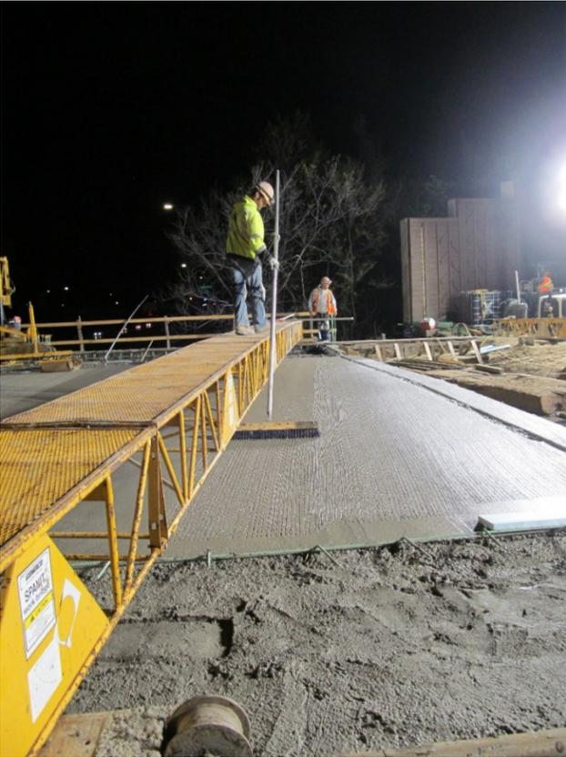
**Figure 2.9: Consolidation and Finishing of IC-LC-HPC-4 Sidewalk Sections**
