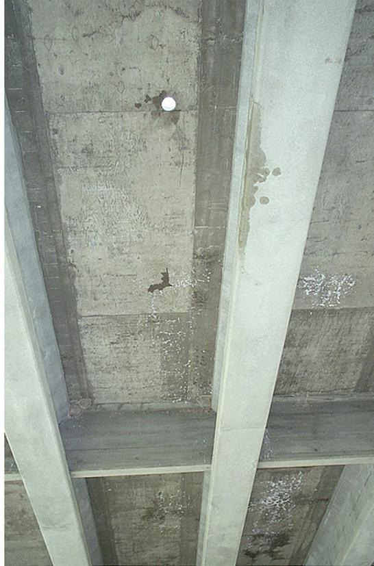
Figure T-3: Photograph from beneath bridge deck after coring operation. Hole from core T-2 is visible. Dampness permeating through cracks visible beneath the area of core T-1. White efflorescence common in areas directly below regions covered with cold patch material.
