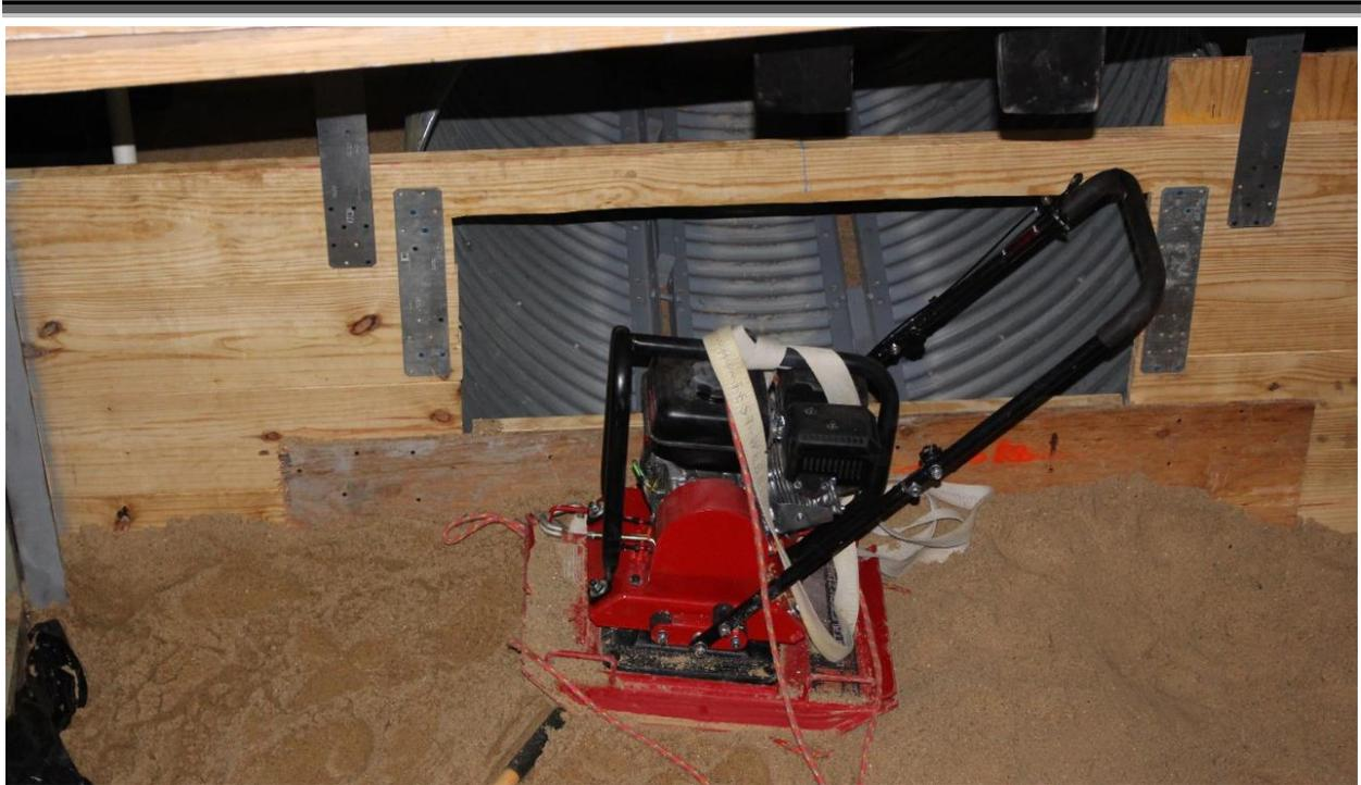
Figure A5: Vibratory Plate Compactor
