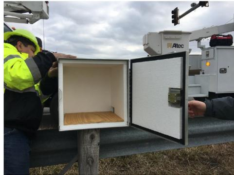
A box for mounting the field monitoring system
