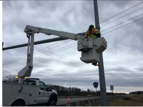
Replacing with the new self de-icing signals
