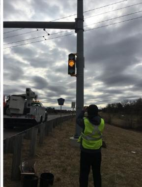
New green /orange signals are powered on
