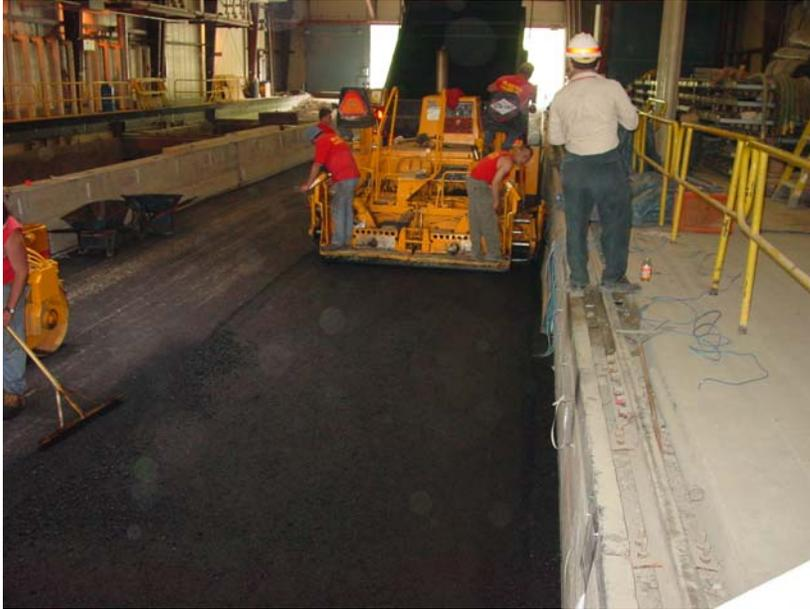
**Figure 27. Image of paving operation during placement of the surface course of asphalt. The dump truck containing the asphalt concrete is in the background and the paver is shown in the middle.**
