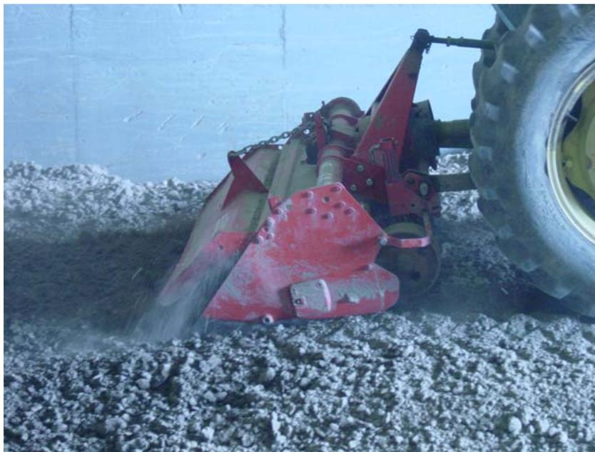
**Figure 15. Cultivating the soil to facilitate moisture absorption and uniform distribution.**
