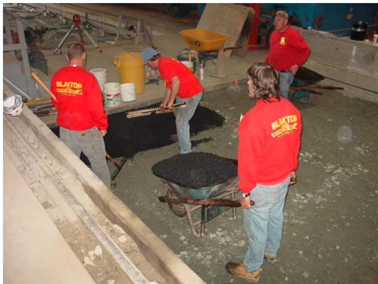
**Figure 26. Hand placement of asphalt near north edge of test basin.**
