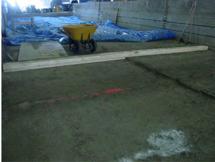
**Figure 18. Image showing differences in elevation of the top of the subgrade between test sections.**
