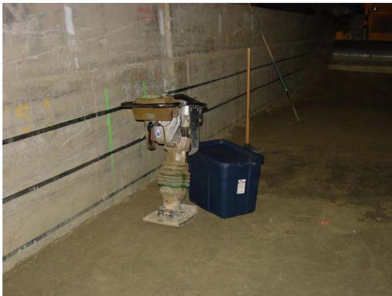
**Figure 16. Plate compactor used to compact the edges of the test section.**
