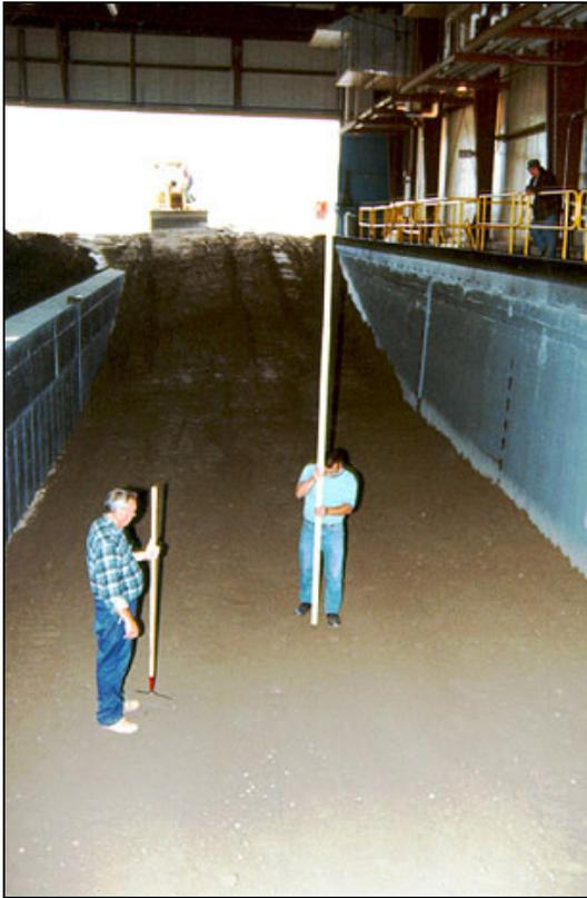
**Figure 23. Rod and level measurements taken on the compacted subgrade lift.**
