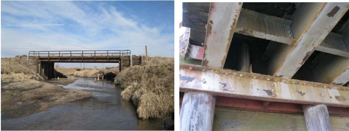
**Figure 3. A representative steel-timber bridge**
