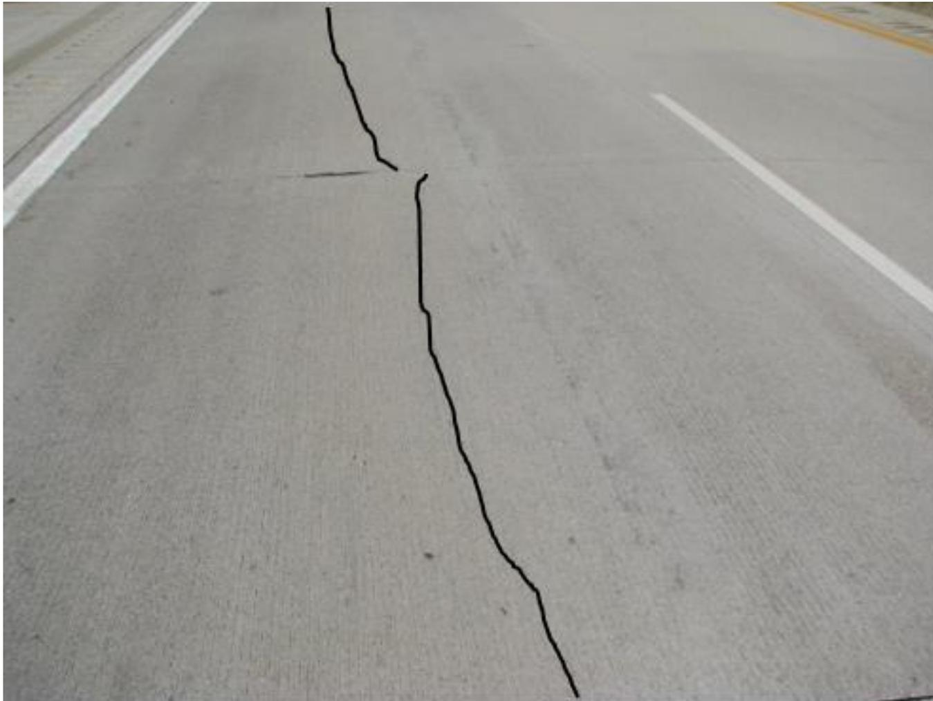
Longitudinal cracks on US 10 near Coleman
