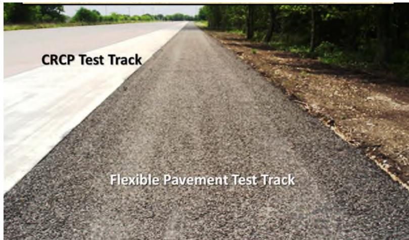
Figure 4.2. New test tracks at the TTI Riverside Campus (Fernando, 2013).
