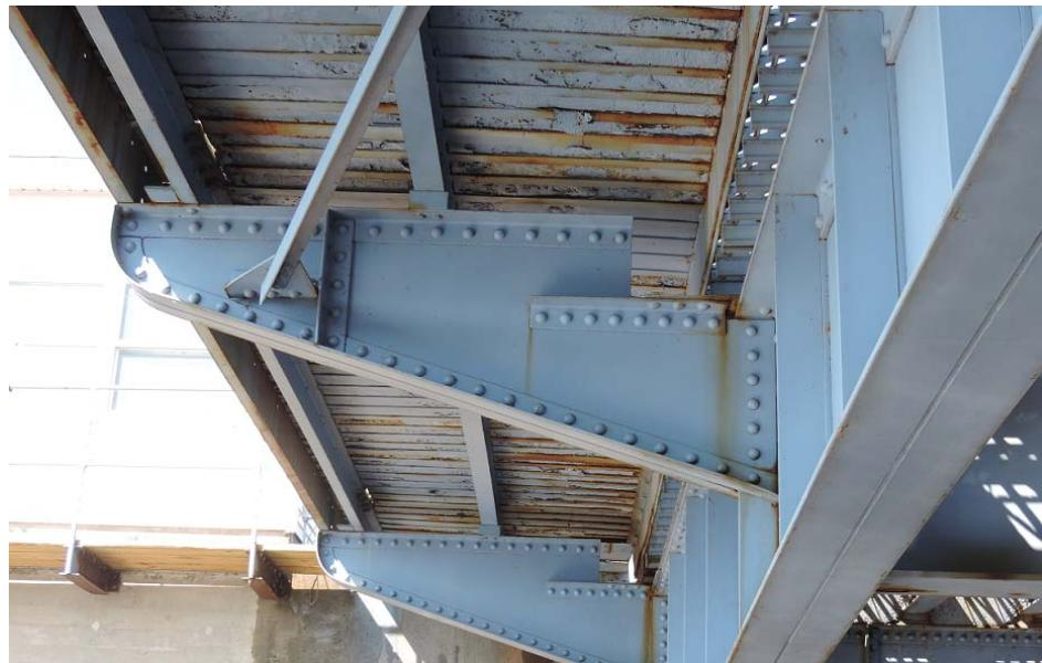
**Figure 5.2-2.** Sidewalk cantilevered on brackets connected to girder web.
