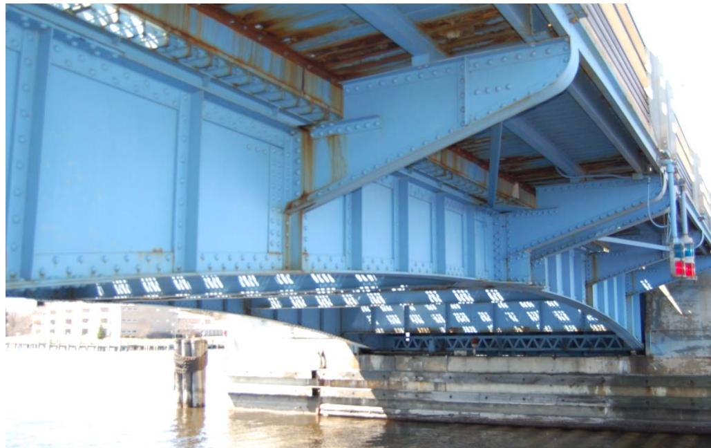
**Figure 5.1-3.** Bascule Girder view. Stiffeners every 3.6 ft. and a variable cross section along the bridge.
