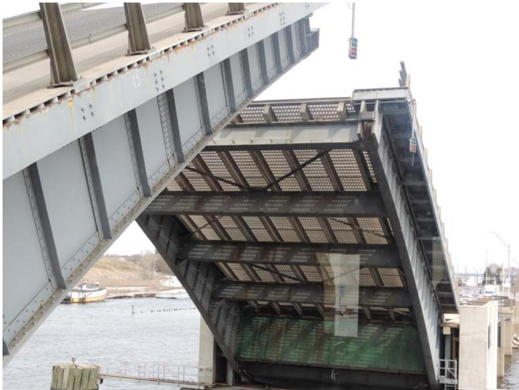
**Figure 4.1-4.** View of Marinette framing from below leaf and joint locking mechanism at the open end of the bascule girder.
