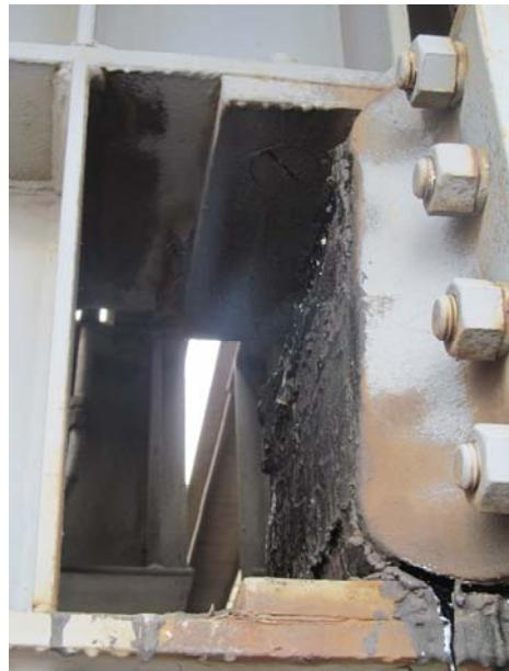
**Figure 4.2-14.** Joint between leaves of Marinette bascule bridge.
