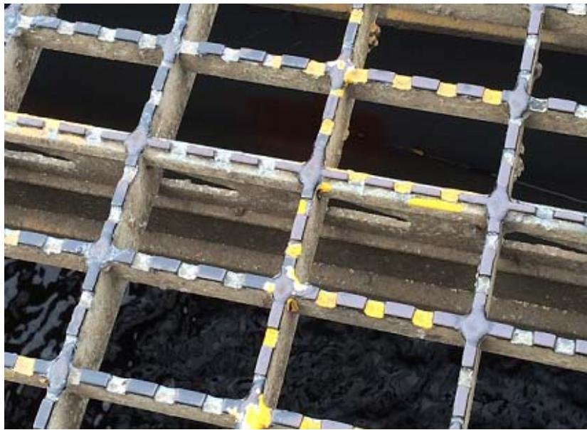
**Figure 4.1-5.** 5-in. steel open welded grid flooring.
