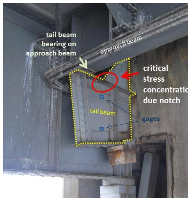
**Figure 4.2-9.** Tail beam region with bearing and notch.
