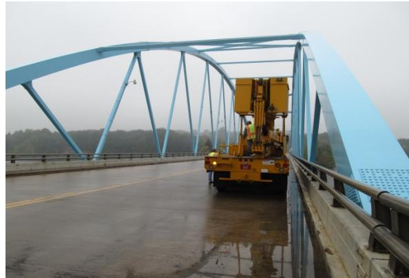
**Figure 7.1-3.** Chippewa bridge deck during inspection in 2013.
