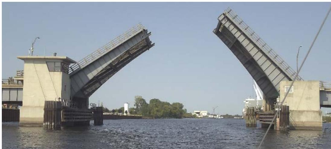
**Figure 4.1-2.** Marinette Bridge (Wisconsin, HIS ID: B38016, Bascule bridge, span = 143 ft.).
