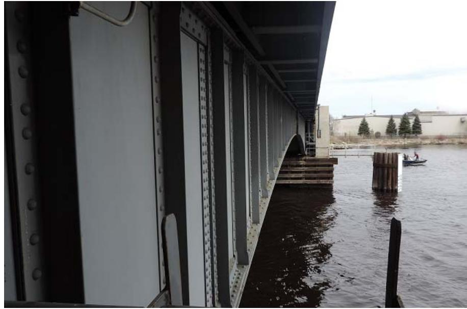
**Figure 4.1-5.** Bascule Girder view. Stiffeners every 3.5 ft. and a variable cross section along the bridge.
