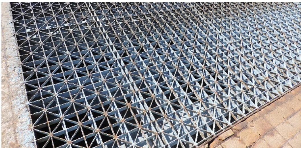
**Figure 5.1-4.** 5-Inch 4-Way modified open grid metal deck.
