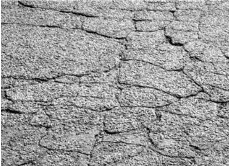
**Figure 1.1 Pavement Showing Block Cracking Distress**
