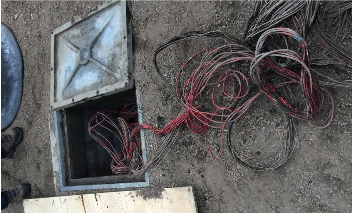
*Figure 2 Sensor wires in pull box*
