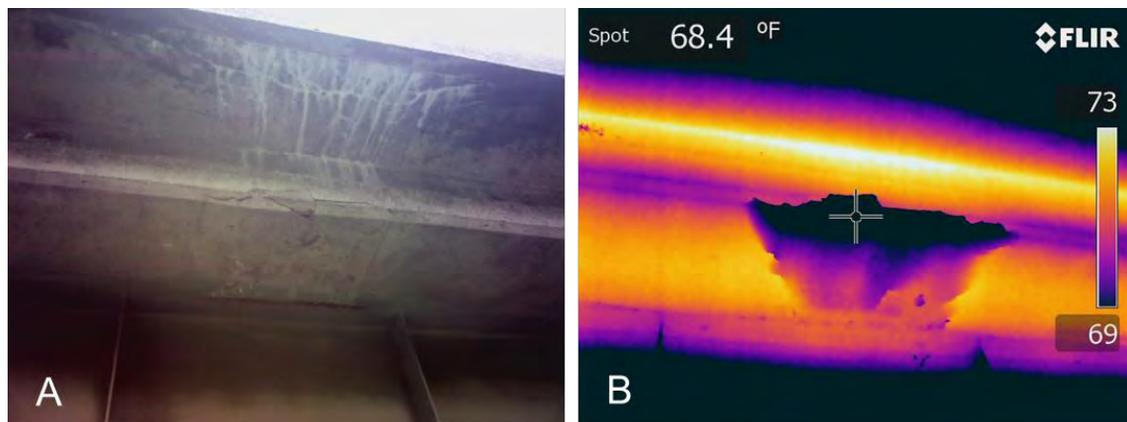
**Figure 13: Images of a delamination along the edge of the bridge**
