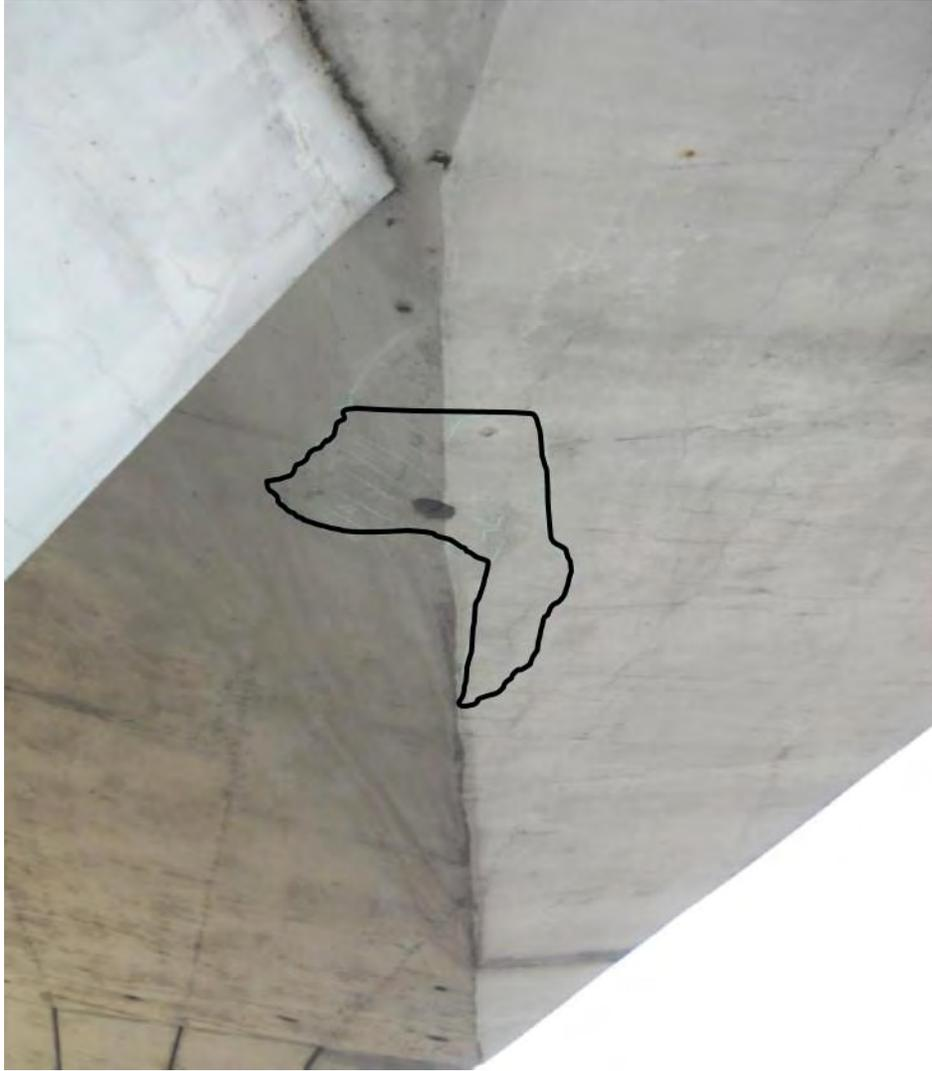
**Figure 36: Hammer sounding results of a drain delamination from the WJE report**
