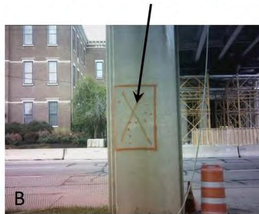
Figure 40: IR (A) and digital (B) images of hammer sounding results on a pier in Kentucky
