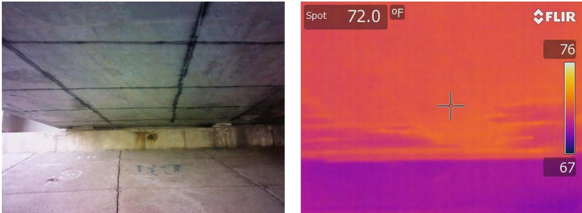
Figure 9: Standard and IR photos of bridge soffit delaminations (Duluth, Minnesota)
