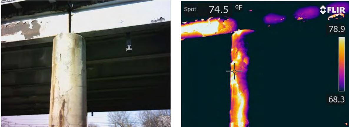
Figure 11: Standard and IR photos of bridge substructure delaminations (Albany, New York)
