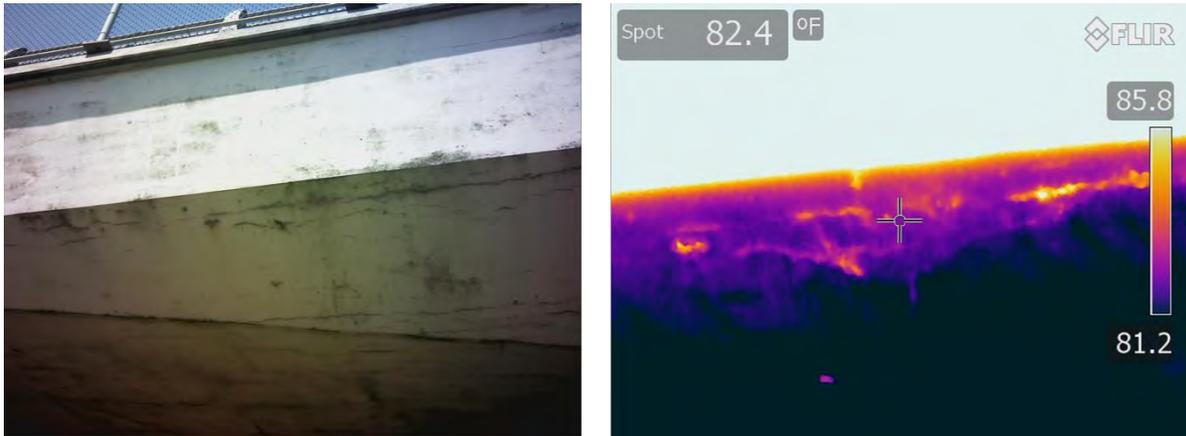
Figure 15: Standard and IR photos of bridge soffit delamination (Woodburn, Oregon)
