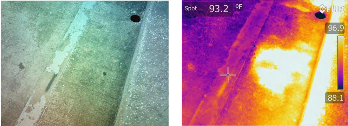
Figure 1: Standard and IR photos of bridge deck delamination (St. Petersburg, Florida)
