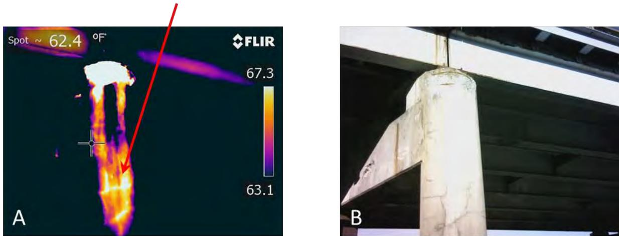
**Figure 43: IR (A) and digital (B) images of a delaminated column on Pier 1 of South Bridge**
