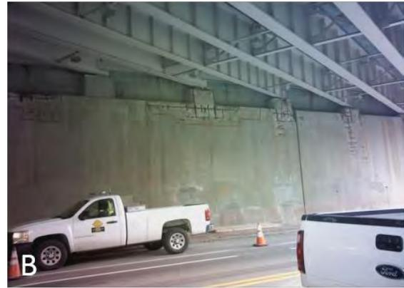
Figure 39: Thermal (A) and Digital (B) images of a delaminated abutment wall under I-265
