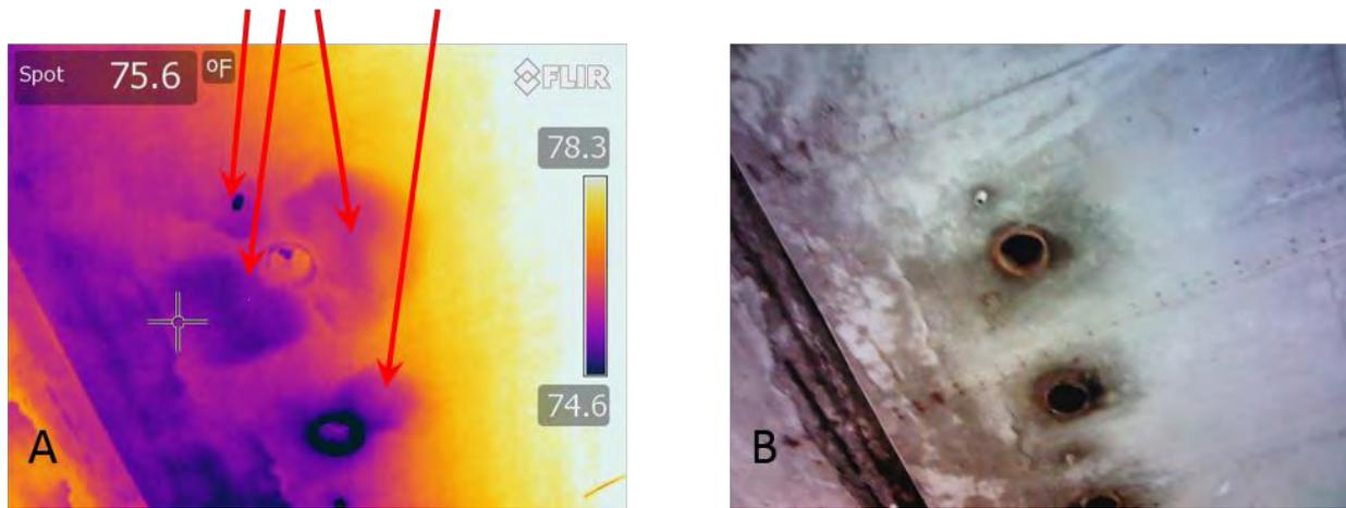
**Figure 48: Morning infrared (A) and digital (B) images of a soffit delamination in Columbus, Ohio**
