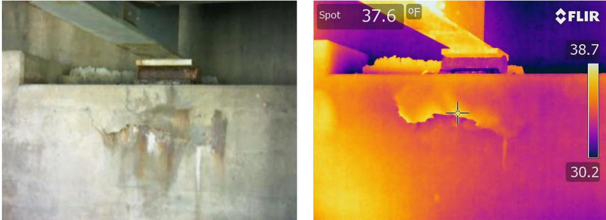
Figure 19: Standard and IR photos of bridge support delamination (Richland Center, Wisconsin)
