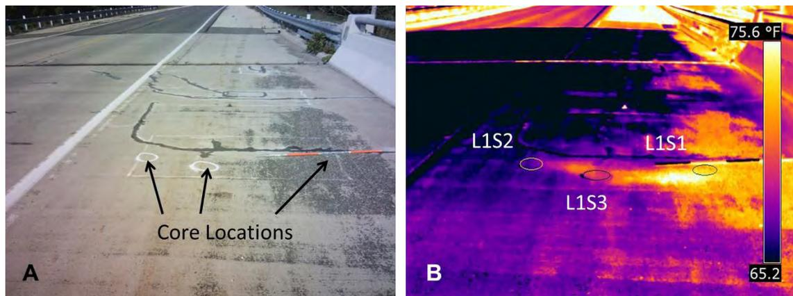
**Figure 10: Cores at Location 1**
