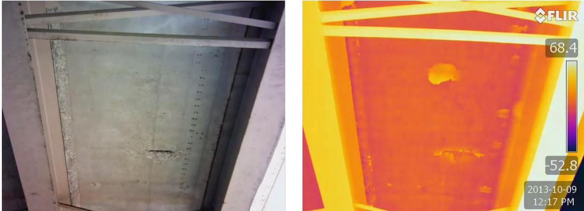
Figure 13: Standard and IR photos of bridge substructure delaminations (Harveysburg, Ohio)
