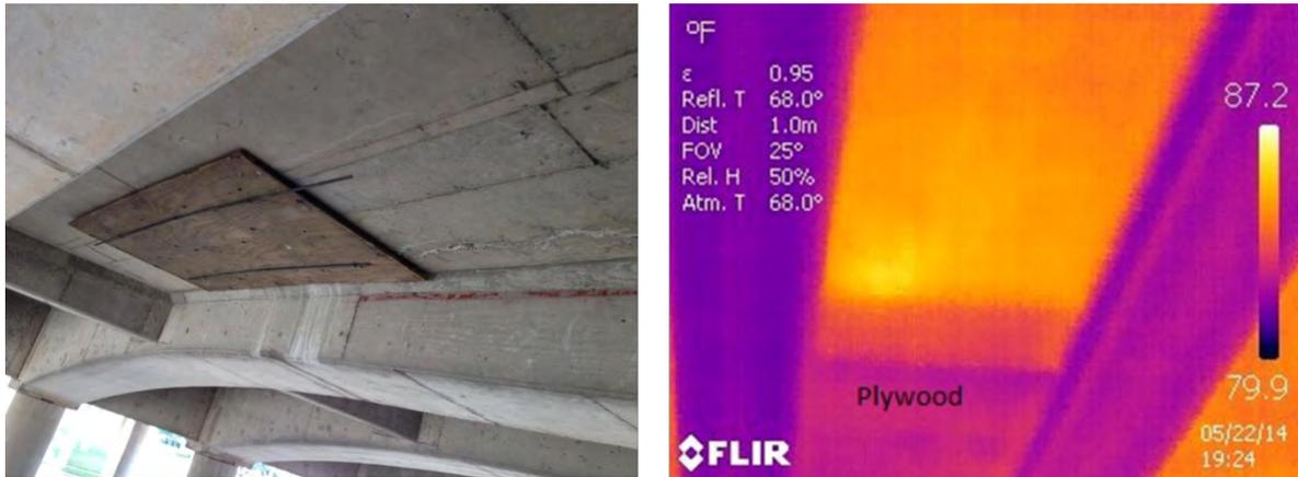
Figure 17: Standard and IR photos of bridge soffit (Waco, Texas)
