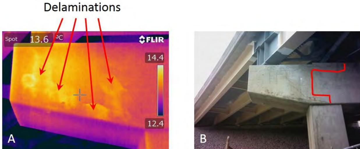
**Figure 31: Thermal image (A) and digital image (B) of a pier cap delamination**
