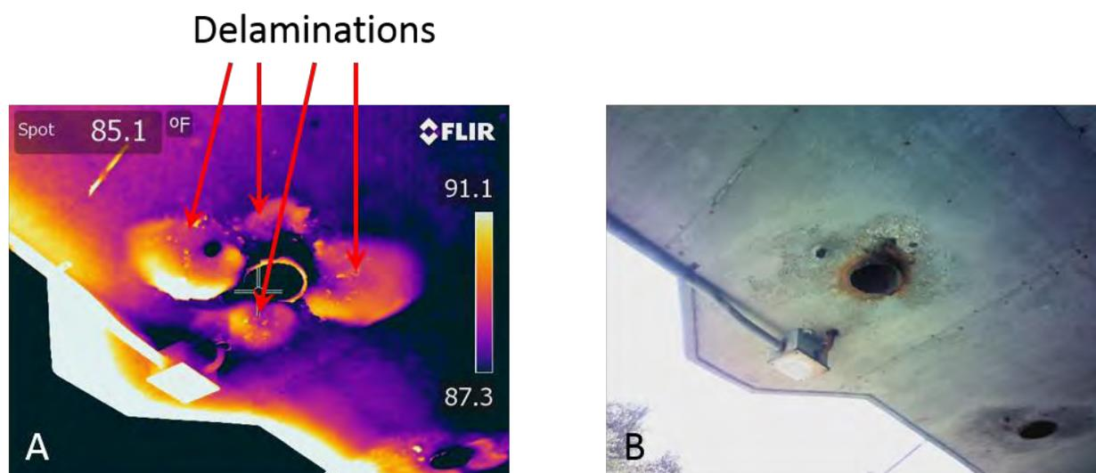
**Figure 47: Afternoon infrared (A) and digital (B) images of a soffit delamination in Columbus, Ohio**
