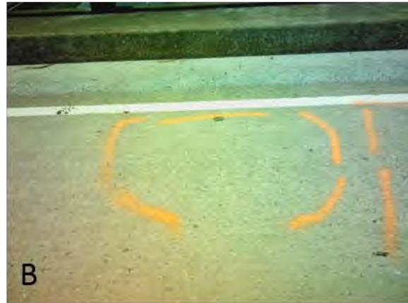
**Figure 27: IR (A) and digital (B) images of a deck delamination on Johnstonville Rd.**
