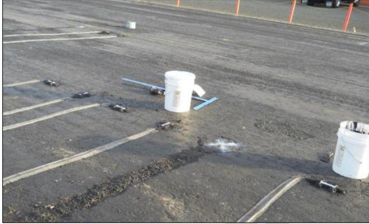
Figure F-13. View of strain gauges and pressure cells installed on Section 670HC during construction.
