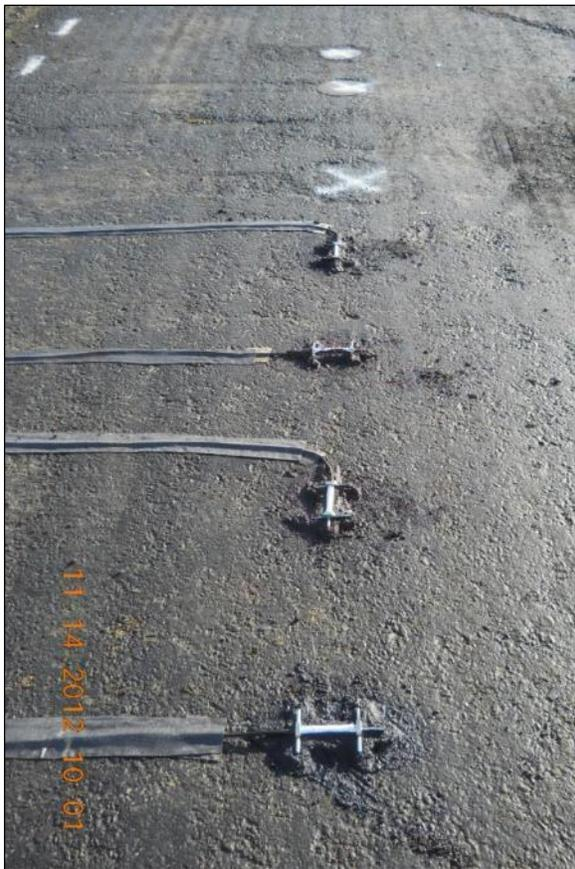
(a) Instruments on top of the recycled base
