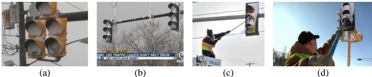
**Fig. 1** Snow-clogged “cool” LED traffic lights and their cleaning off by hand<sup>[3, 4]</sup>
