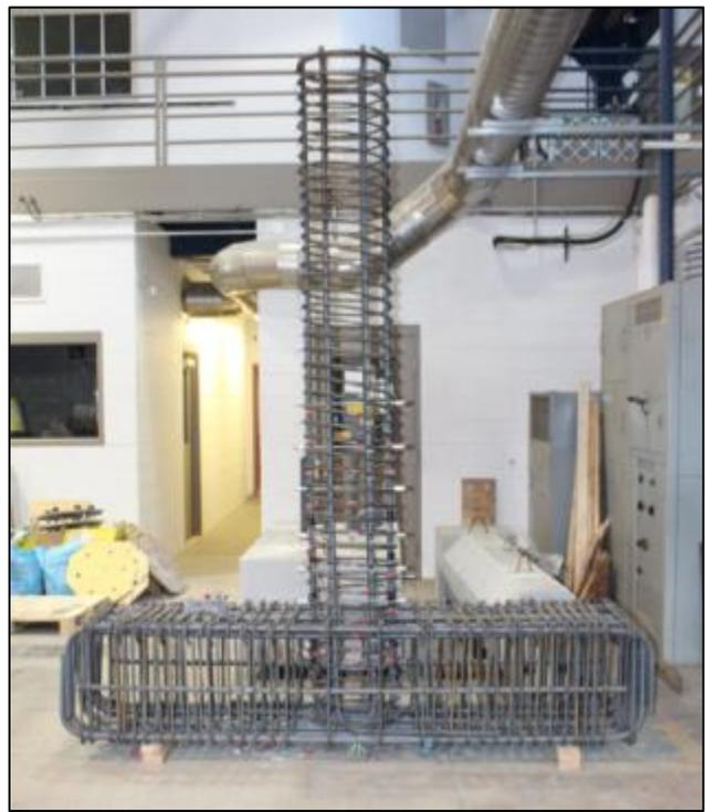
(b) Rebar cage ready to cast concrete.
