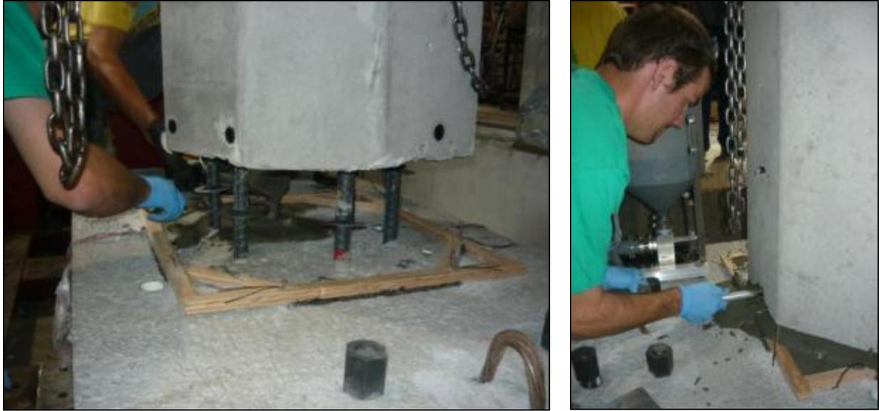
Figure 2-7. Grouting operation for GGSS-1.
