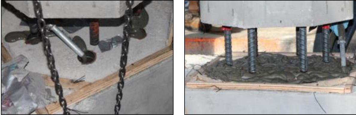
Figure 2-37. Grouting operation for FGSS-2.
