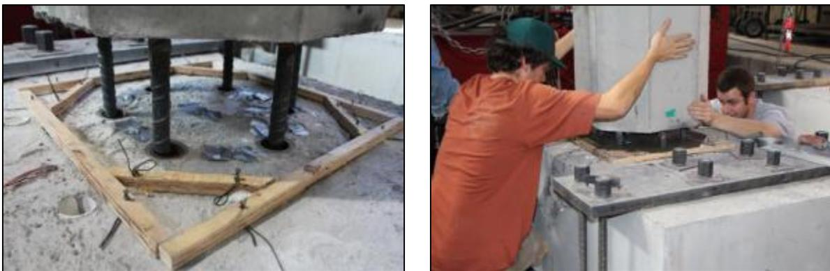
Figure 2-14. Grouting operation for GGSS-2.
