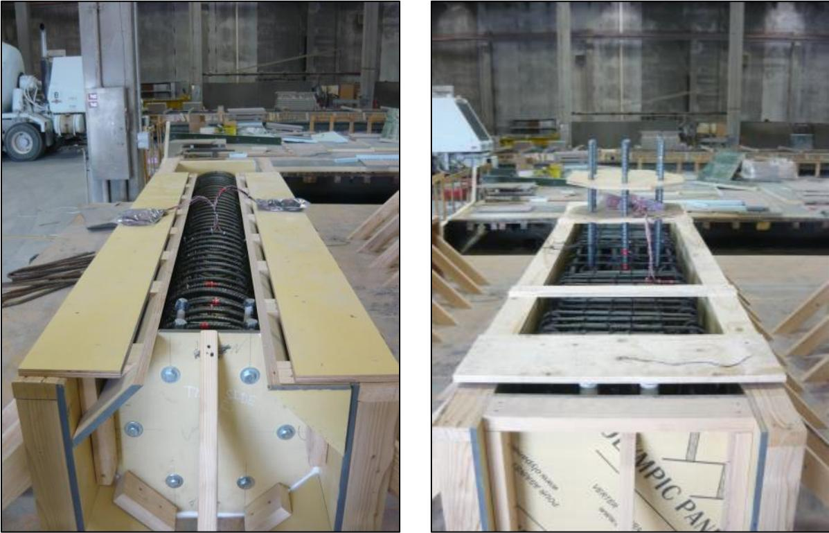
Figure 2-30. FGSS-1 precast components inside concrete forms.
