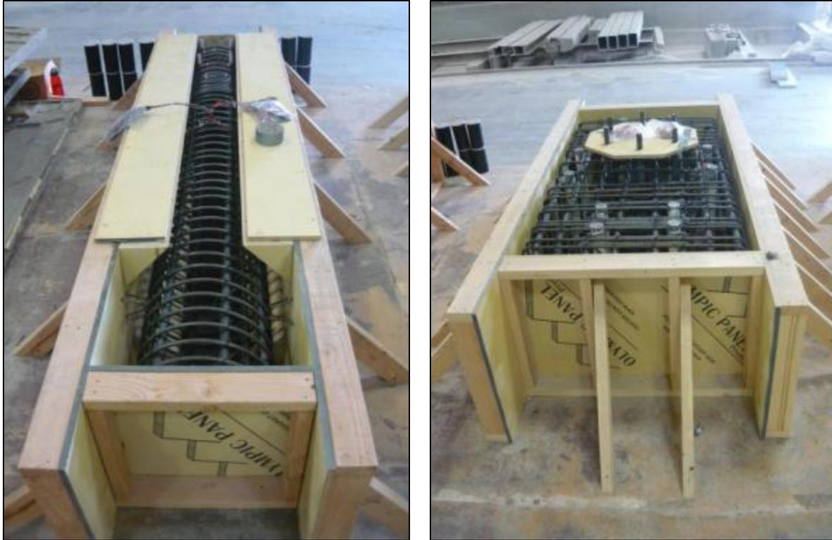
Figure 2-6. GGSS-1 precast components inside concrete forms.
