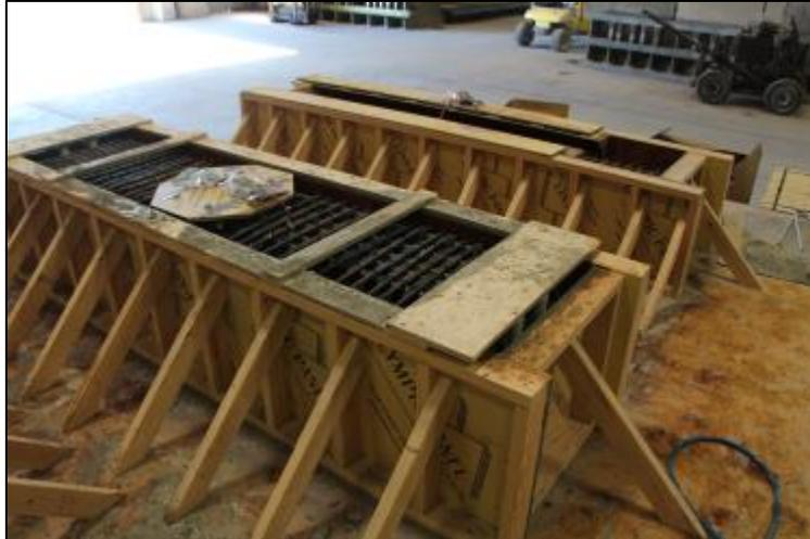
Figure 2-36. FGSS-2 precast components inside concrete forms.
