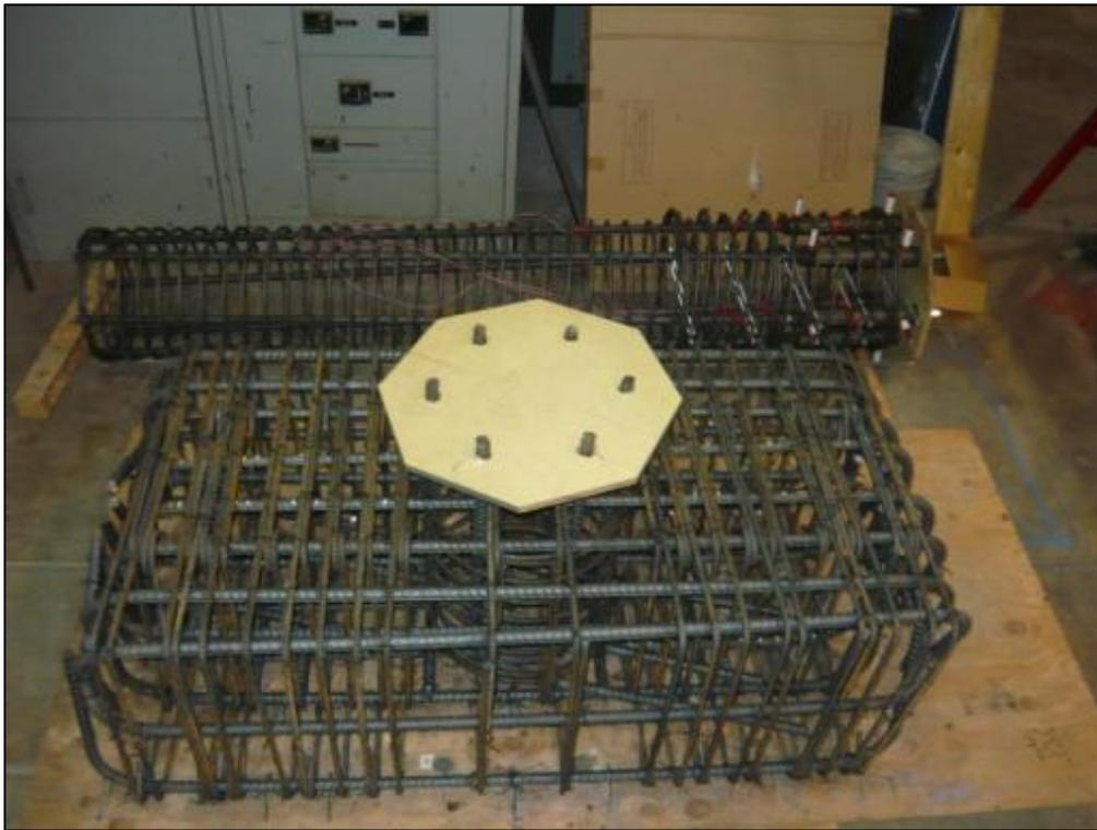
(b) Column and footing rebar cages.
