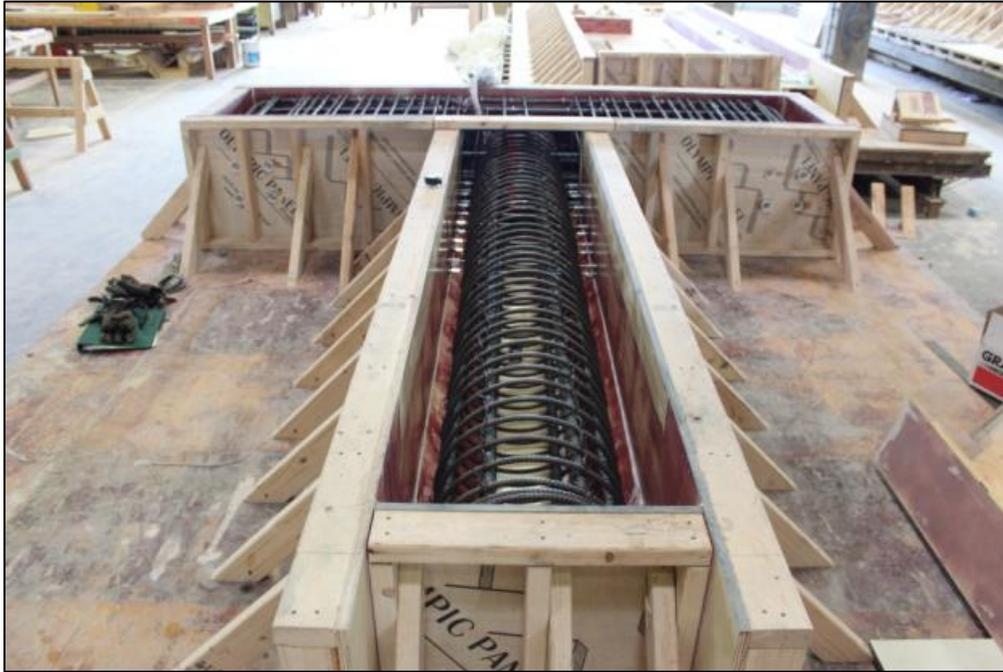
Figure 2-48. FGSS-CIP rebar cage inside concrete form.
