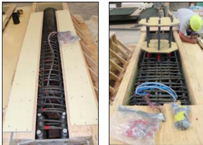
Figure 2-43. FGSS-3 precast components inside concrete forms.
