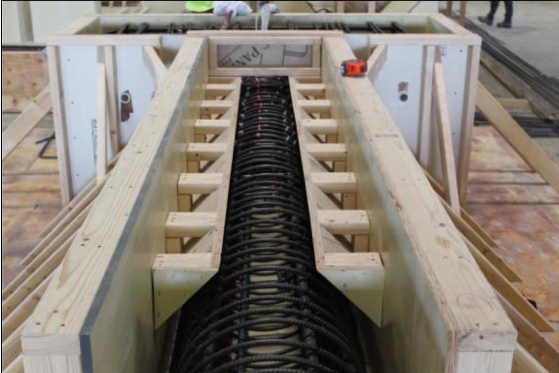
Figure 2-25. GGSS-CIP rebar cage inside concrete form.
