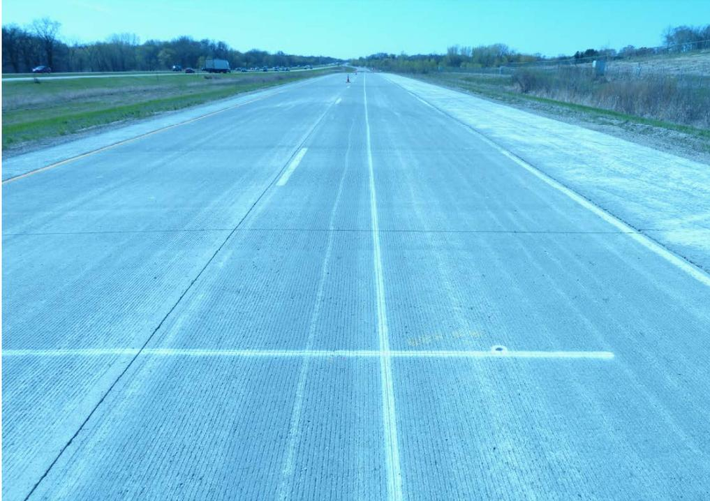
**Figure A-9. Longitudinal tining downstream view.**
