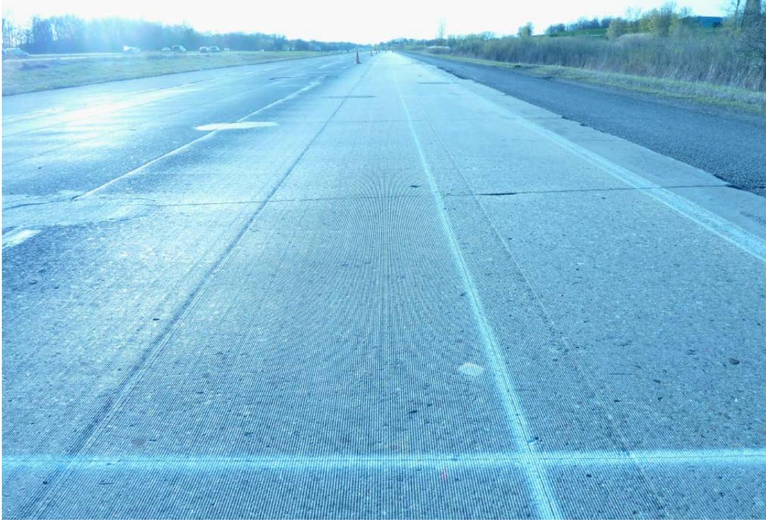
**Figure A-11. Diamond grinding downstream view.**
