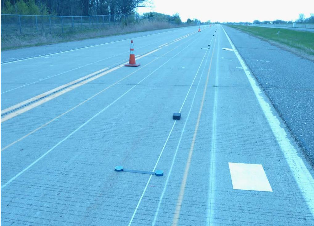
**Figure A-7. Transverse tining downstream view.**
