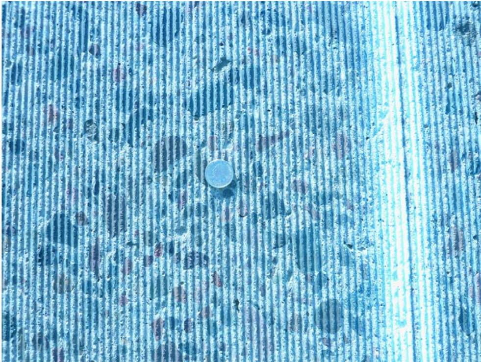
**Figure A-12. Diamond grinding texture.**
