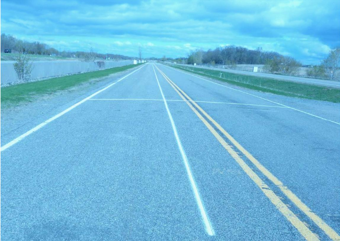
**Figure A-3. Chip seal upstream view.**
