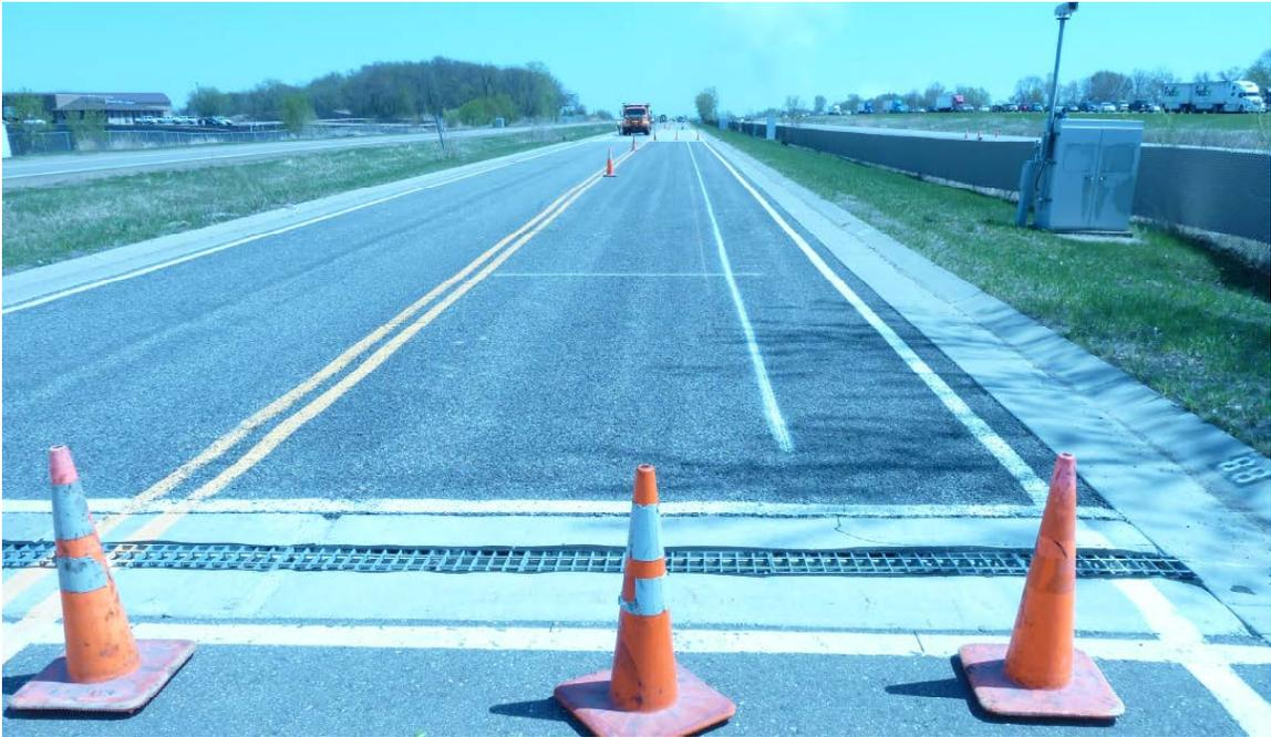
**Figure A-5. Pervious hot mix asphalt downstream view.**
