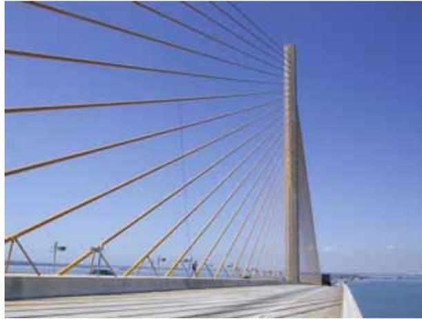
**Figure 26. Photo. Stay and damper brace configuration.**
