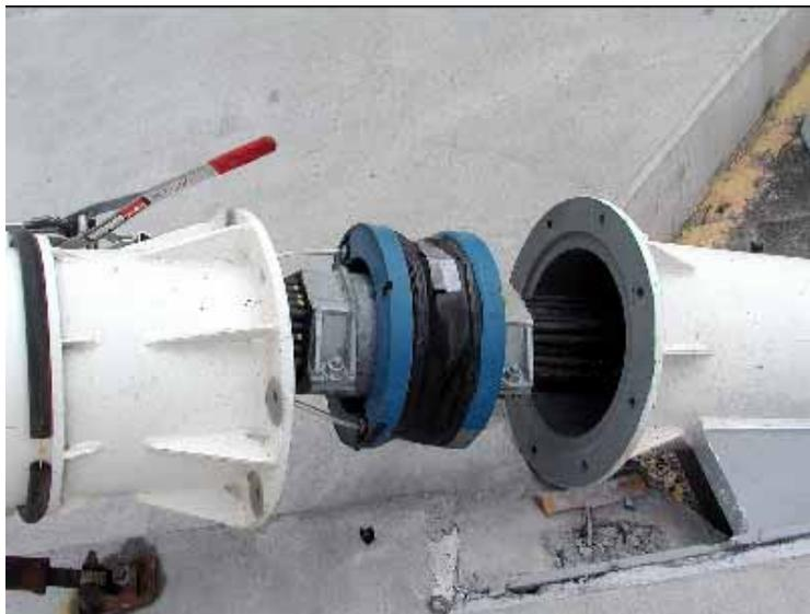
**Figure 6. Photo. Damper at cable anchorage.**
