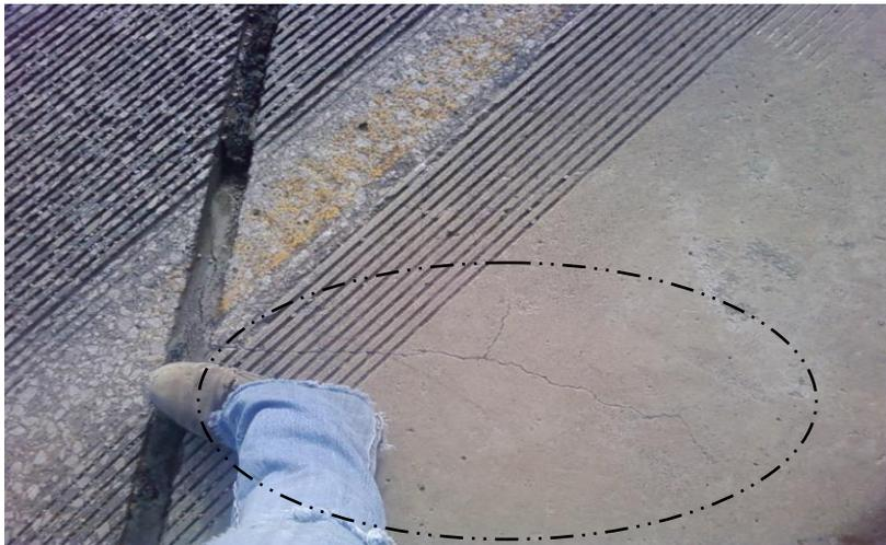
**Figure 4.3. Off-ramp slab cracking**
