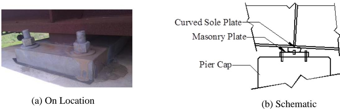
**Figure 5.11. Fixed pier bearing**
