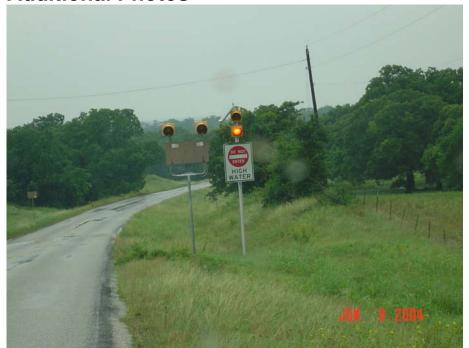
PHOTO #1: Automated warning sign with flashing warning light.
