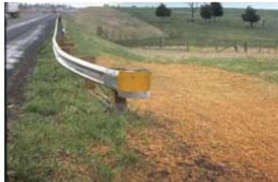
Figure 1-2 Modified Eccentric Loader Terminal (MELT)
