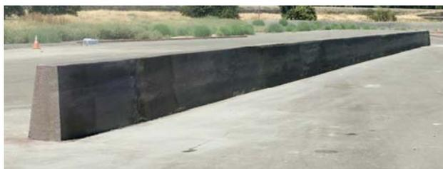
**Figure 2-1 Type 60 Concrete Median Barrier**
