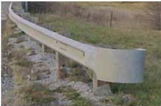
Figure 1-1 Breakaway Cable Terminal (BCT)
