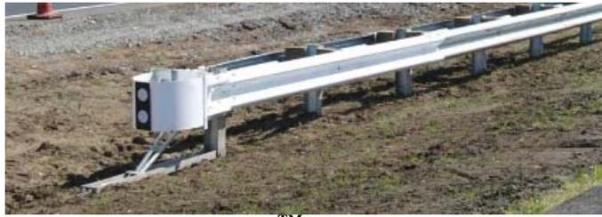
**Figure 4-1 X-Tension™ Guardrail End Terminal**
