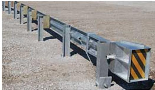
Figure 4-3 Flared Energy Absorbing Terminal (FLEAT™)
