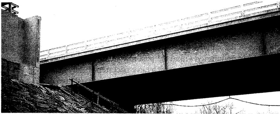
Figure 2. Severe topcoat disbondment.
