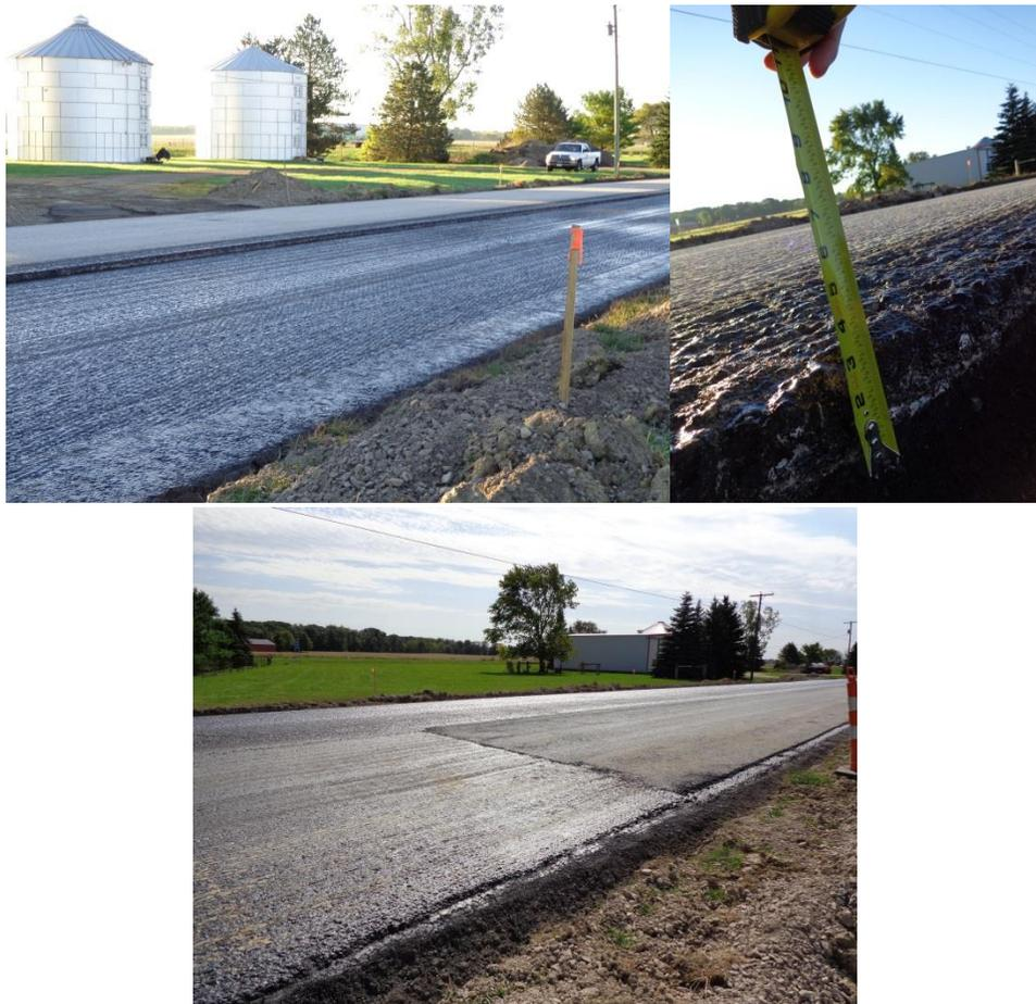
**Figure 38. Milling and fill of ATB in Section A**
