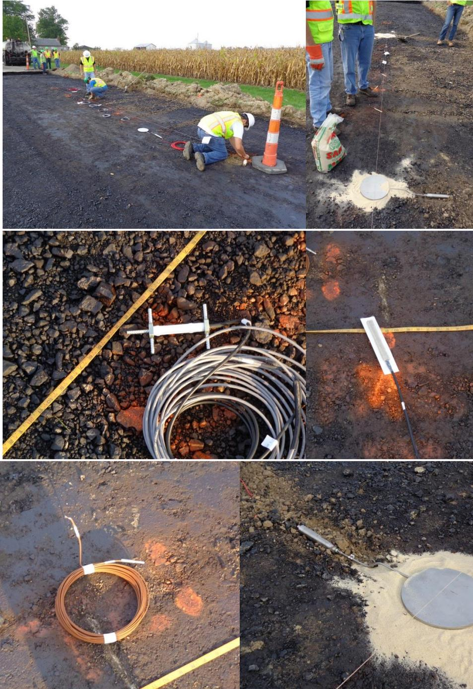
**Figure 28. Instrumentation at the bottom of DGAB in Section A**
