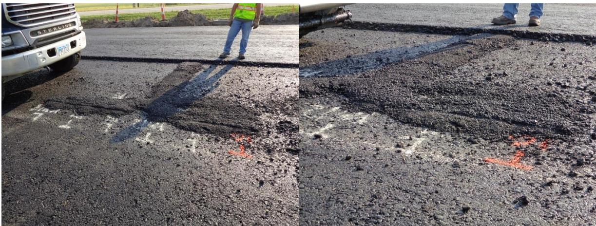
**Figure 34. Possible misalignment of sensors after truck passes**
