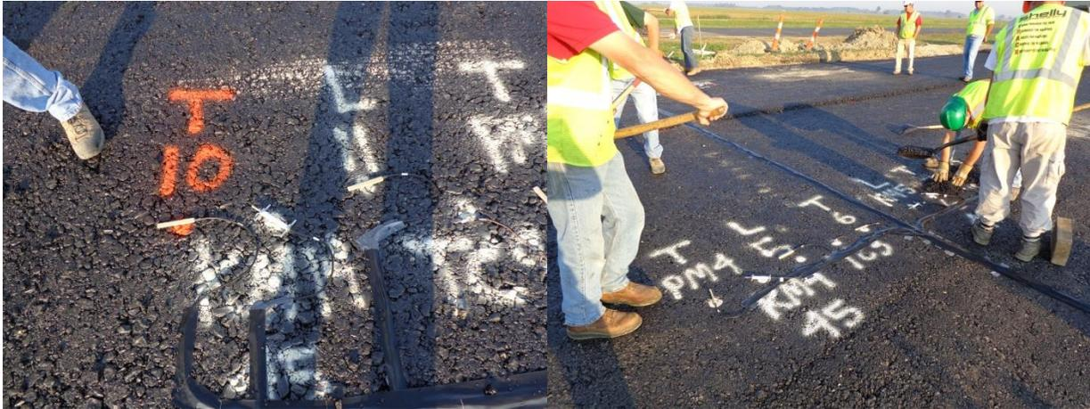
**Figure 33. 45° strain gauge 1 ft apart from adjacent sensors**
