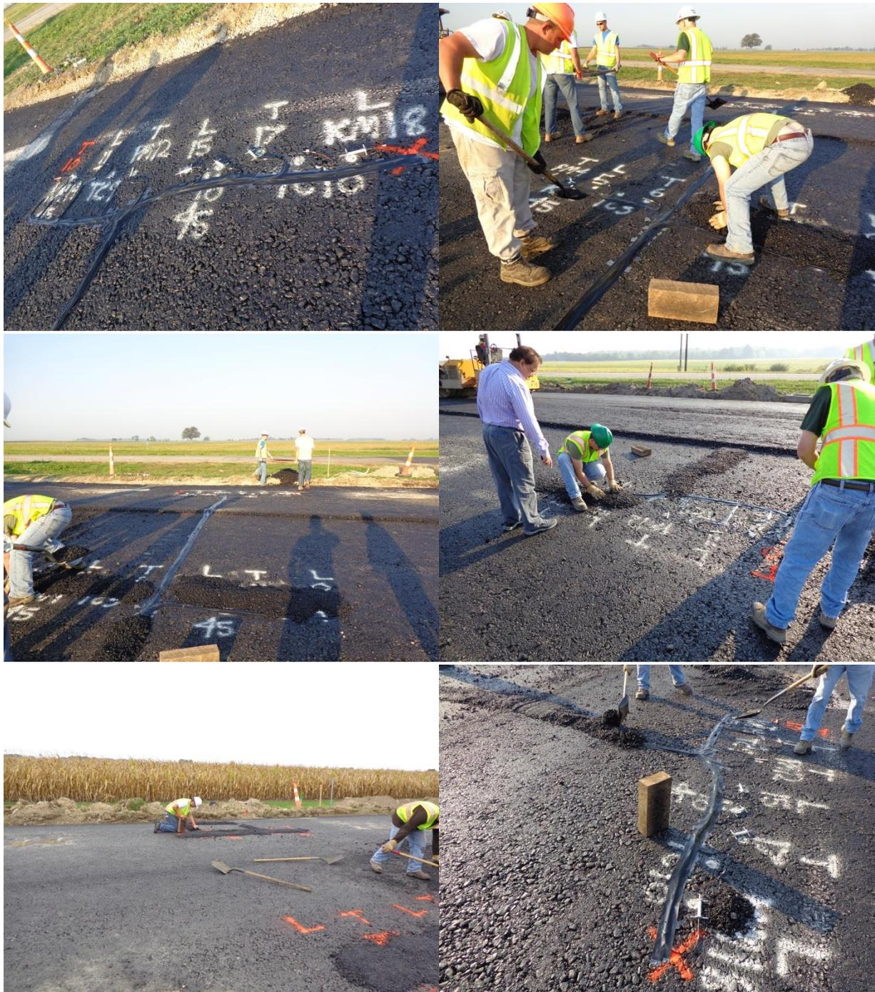
**Figure 32. Instrumentation at the bottom of the ATB**
