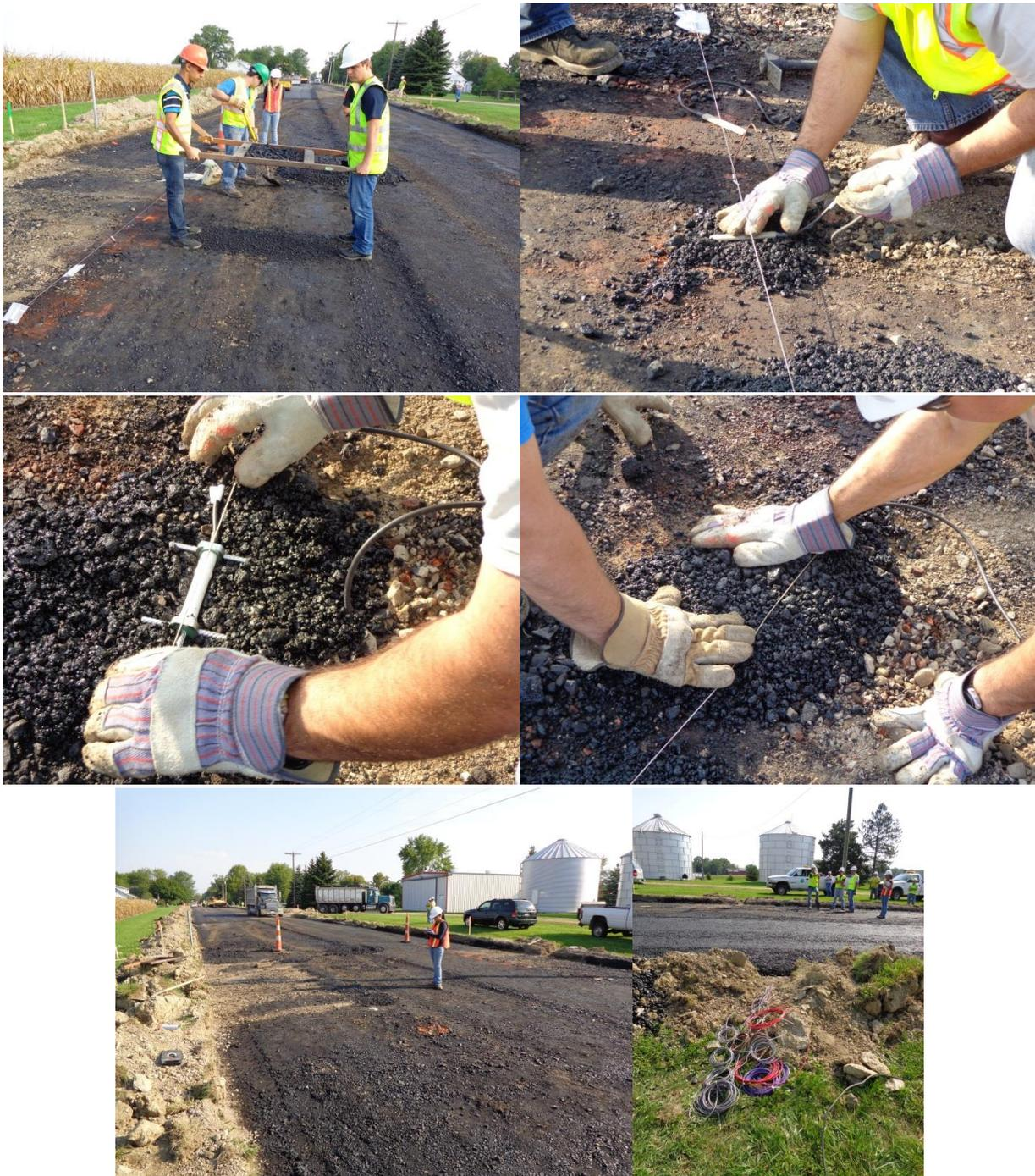
**Figure 29. Installation of sensor at the bottom of the FRL in Section A**
