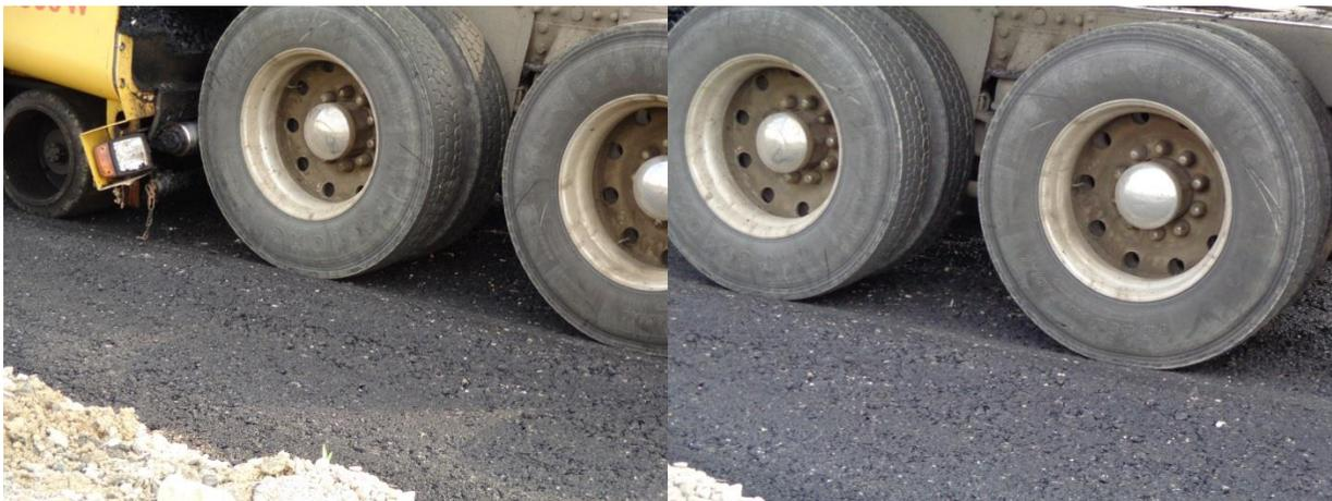
**Figure 35. Rutting of FRL due to weak DGAB**
