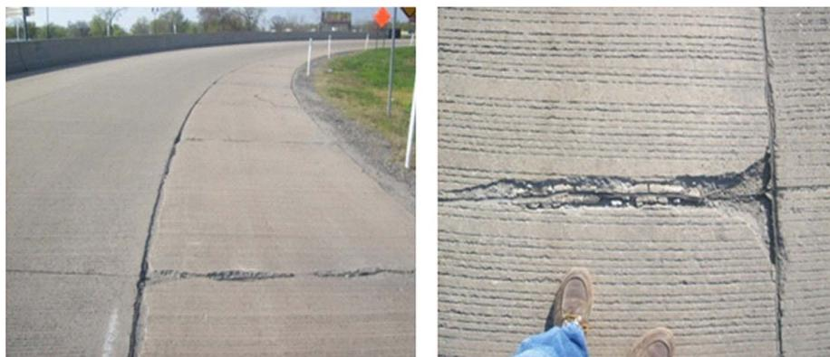
**Fig. 1.** Field observation showing damage in pavement joints
