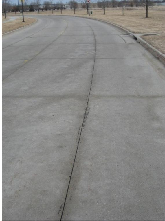
**Figure 4. Wet joints and dry pavement**
