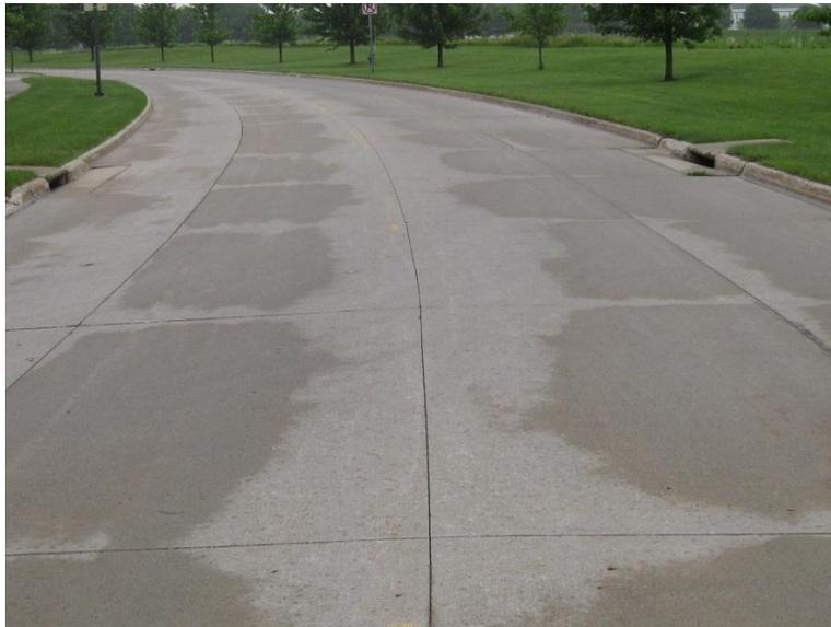
**Figure 1. Evidence of joints that are draining well**
