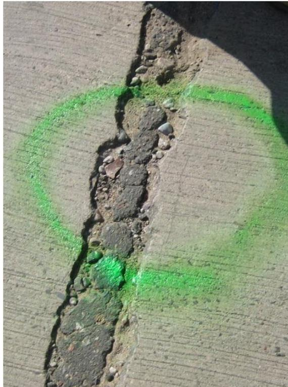
**Figure 1. Crack formed about 1 in. from the free surface**
