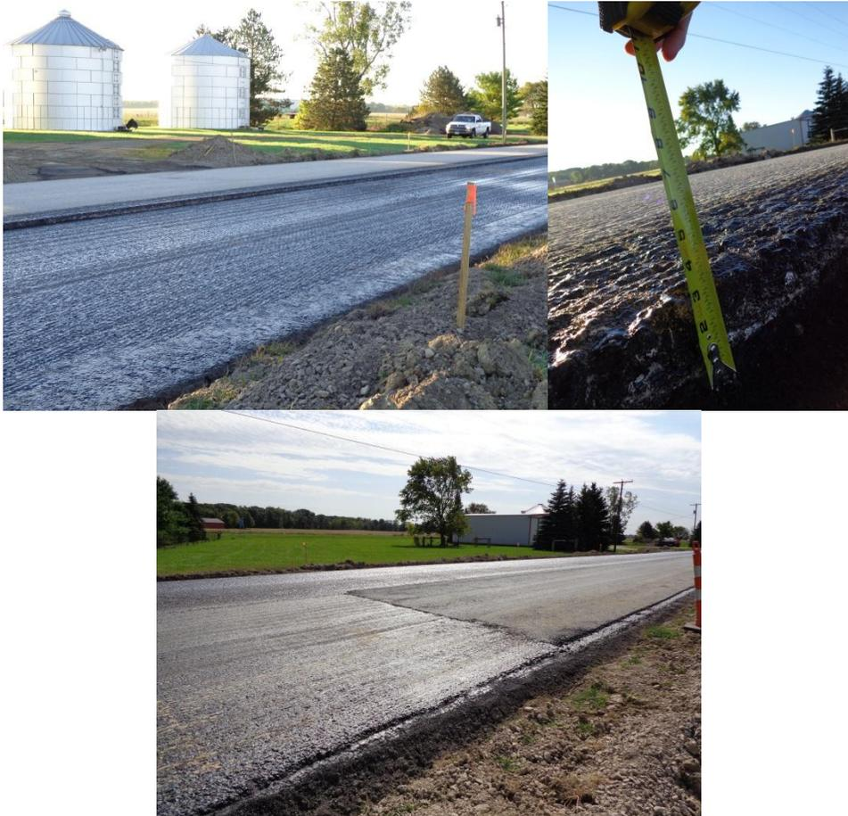
**FigureC-13. Milling and fill of ATB in Section A**
