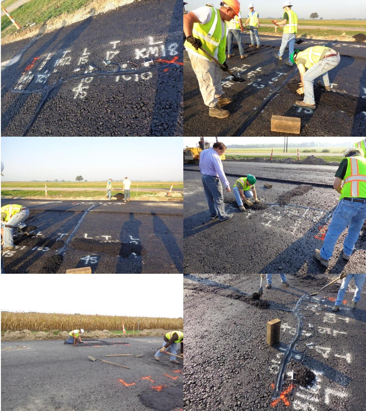
**Figure C-7. Instrumentation at the bottom of the ATB**
