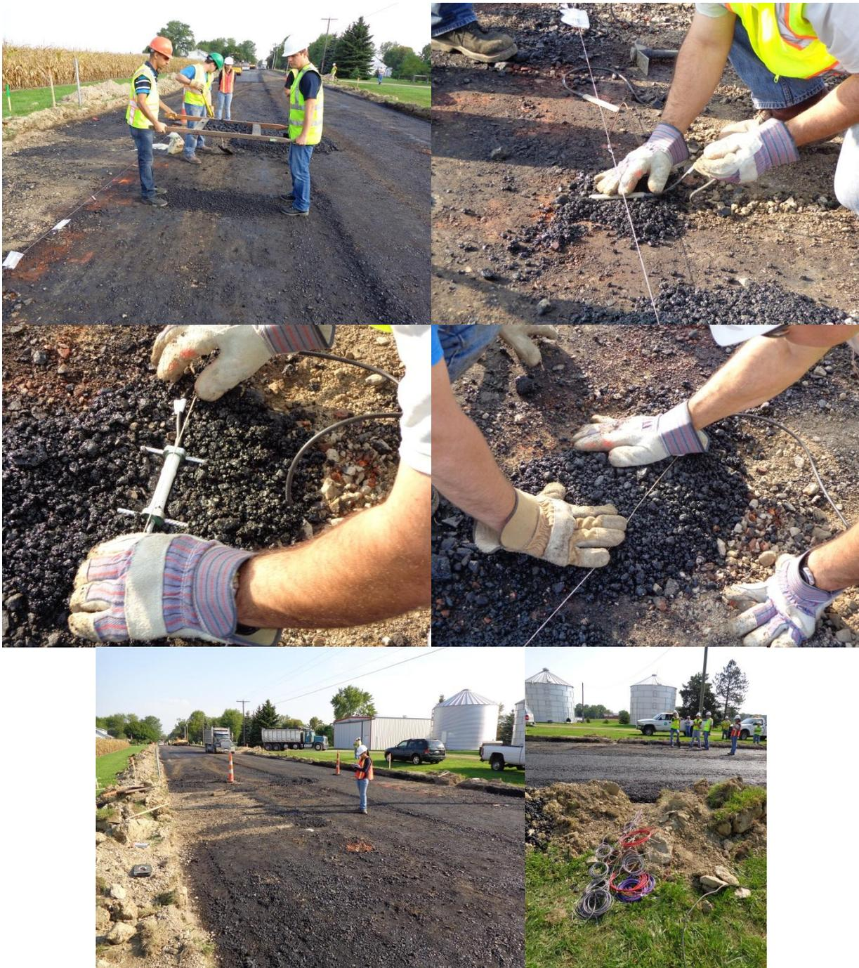
**Figure C-4. Installation of sensor at the bottom of the FRL in Section A**
