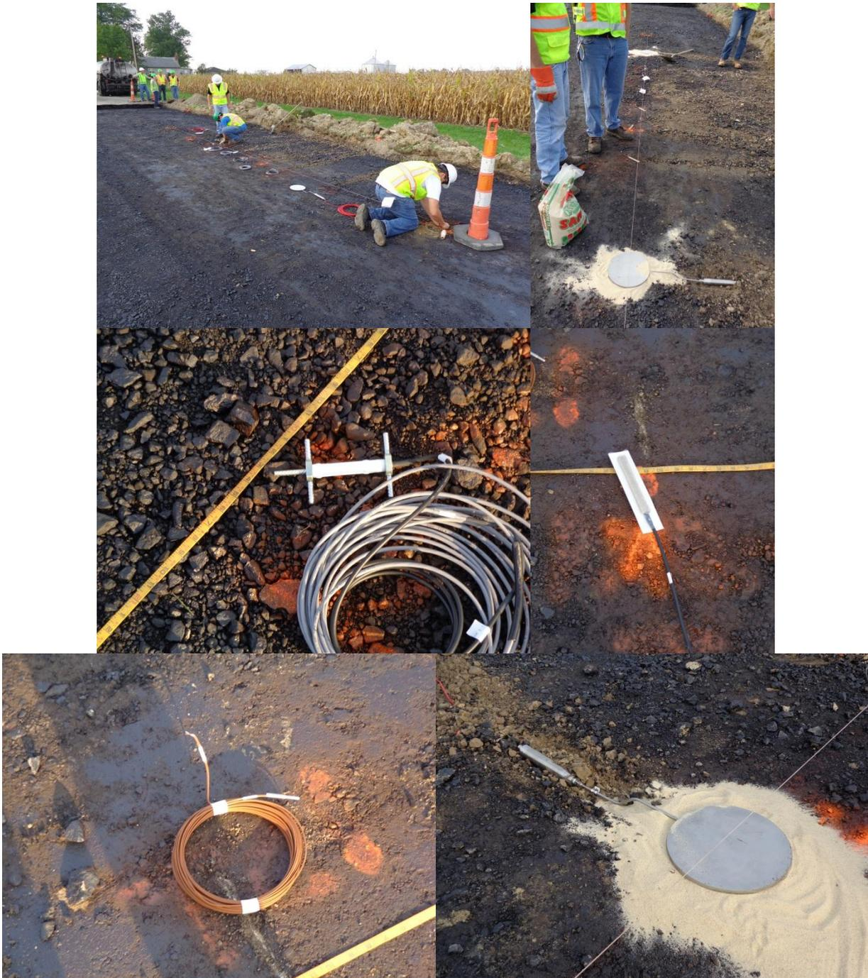
**Figure C-3. Instrumentation at the bottom of DGAB in section A**
