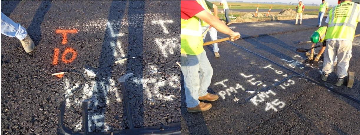
**FigureC-8. 45° strain gauge 1 ft apart from adjacent sensors**
