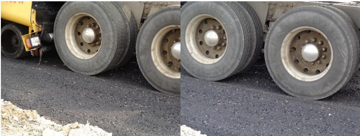
**FigureC-10. Rutting of FRL due to weak DGAB**
