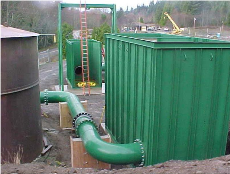
Figure 3. Photograph of Head Water and Tail Water Tanks, December 2002. The test be support and culverts to be tested will be installed between the two tanks. Skookumchuck Hatchery is in the background.
