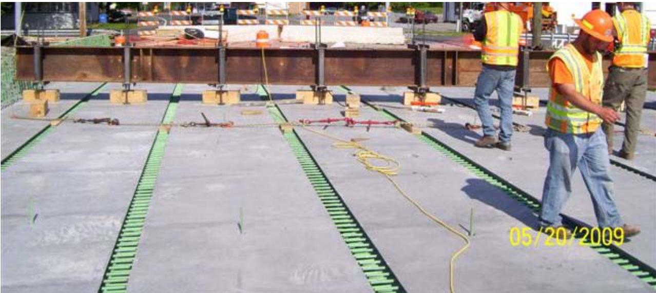
**Figure 1. Photograph. Longitudinal connections prior to field-casting of UHPC in Route 31 Bridge in Lyons, New York. (Photo courtesy of NYSDOT.)**
