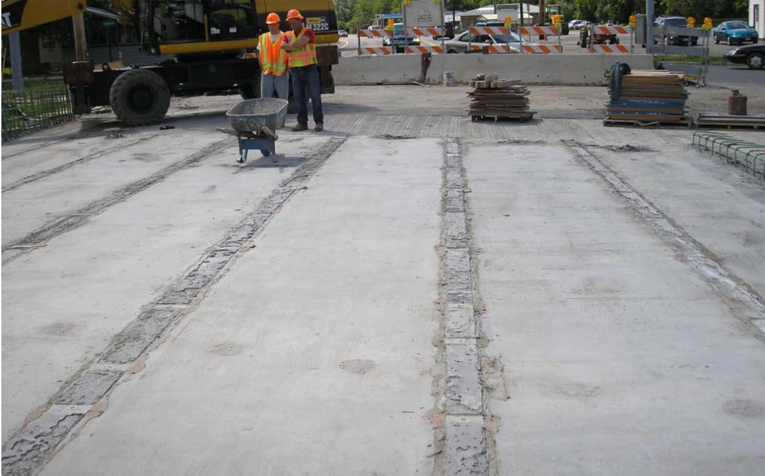
**Figure 3. Photograph. Longitudinal connections after field-casting of UHPC in Route 31 Bridge in Lyons, New York. (Photo courtesy of NYSDOT.)**
