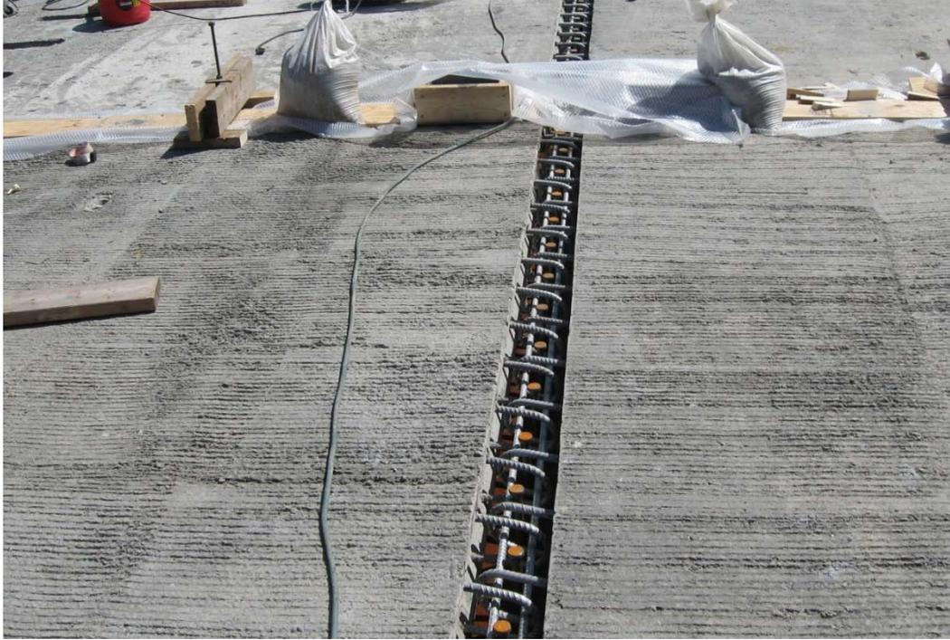
**Figure 5. Photograph. Transverse connectin prior to field-casting of UHPC in Route 23 Bridge in Oneonta, New York. (Photo courtesy of NYSDOT.)**
