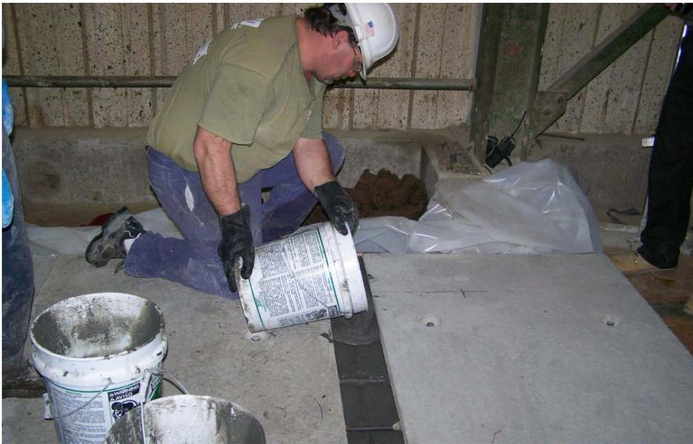
**Figure 13. Photo. Placement of UHPC into connection. (Photo courtesy of NYSDOT)**
