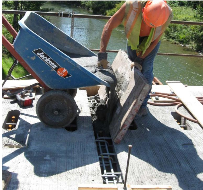
**Figure 6. Photograph. Field-casting of UHPC for Route 23 Bridge in Oneonta, New York.**
