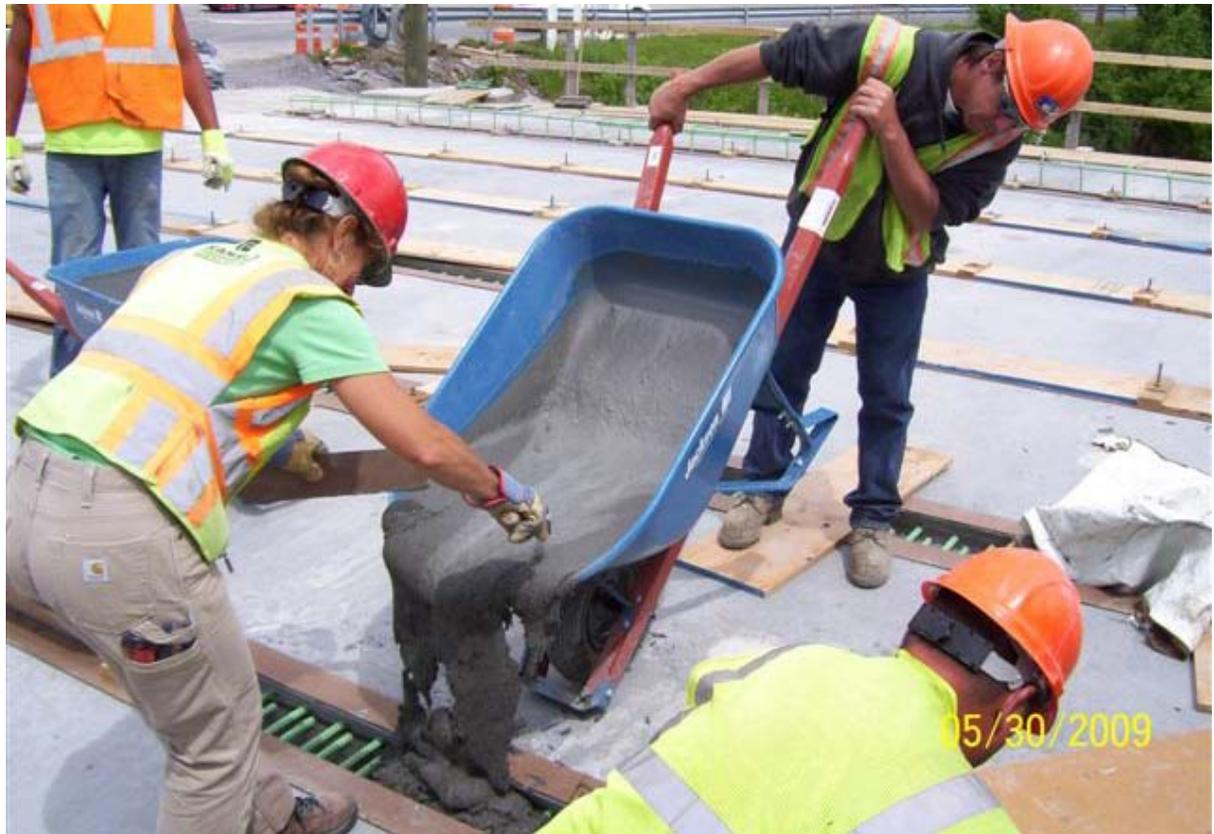
**Figure 2. Photograph. Placement of UHPC into longitudinal connections between deck-bulb-tee girders in Route 31 Bridge in Lyons, New York. (Photo courtesy of NYSDOT.)**
