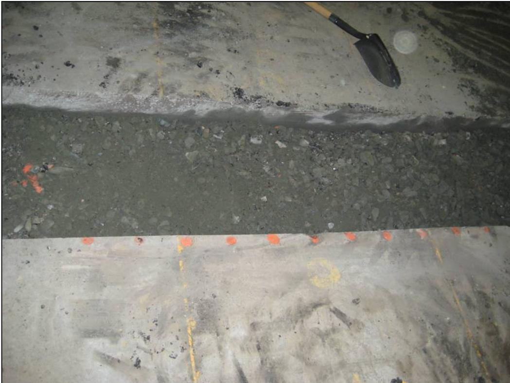
Figure B30. Trench for measuring emu coil distances and soils properties after removing the AC layer.
