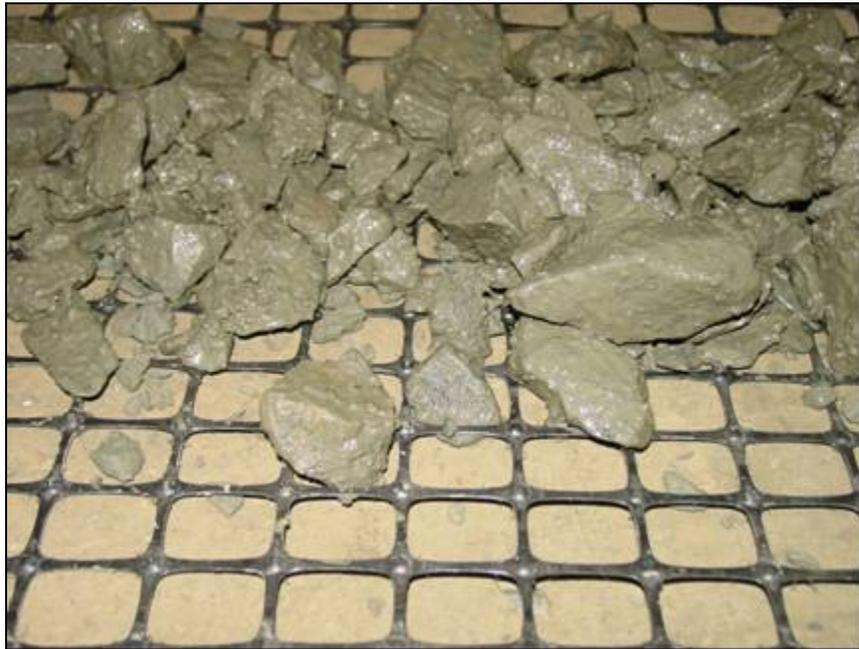
Figure 1. Close-up of Geogrid and base aggregate particles during construction. Aggregate particles protruding partly through the grid apertures suggest good inter-locking.
