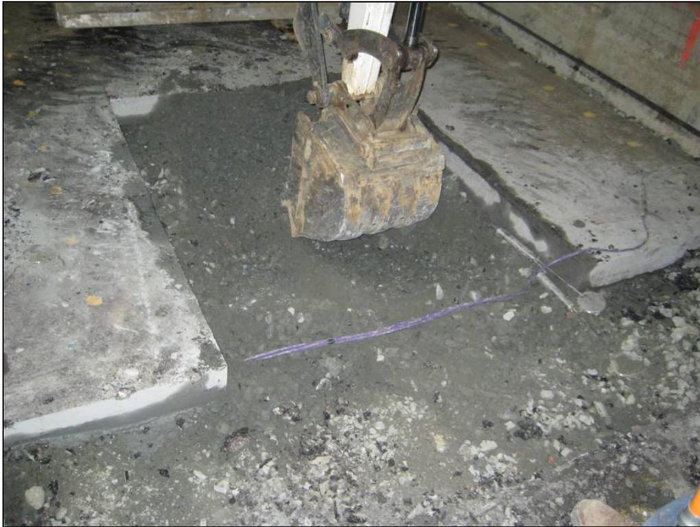
Figure B25. Mini excavator removing base course in TS 7.
