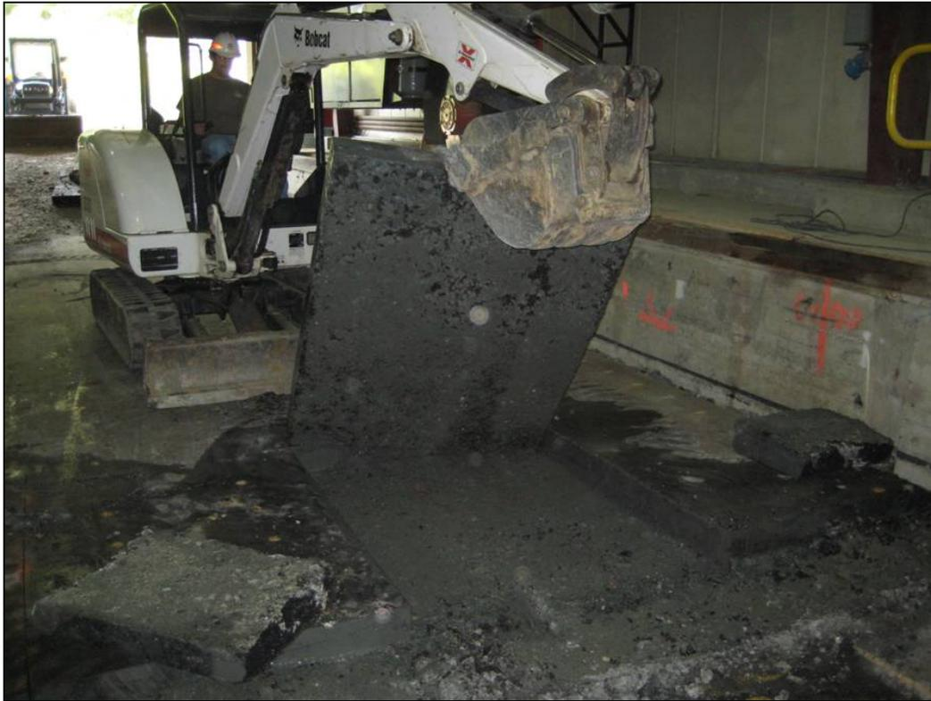
Figure B24. Mini excavator removing a section of the AC layer in TS 7.
