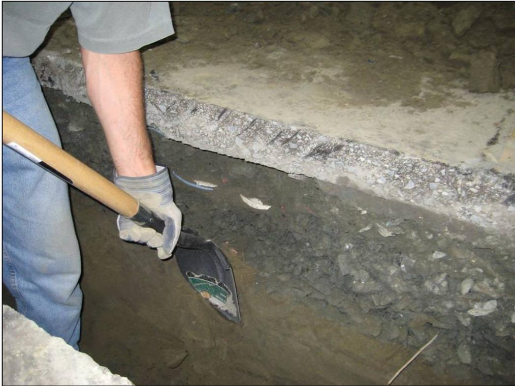
Figure B31. Starting to expose the emu coils in TS 2 using hand tools figure.
