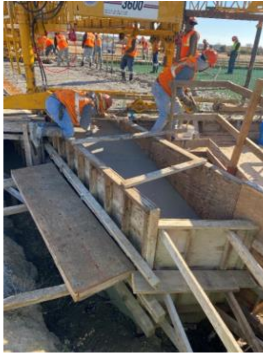
Figure 2.51: Walking Observed on Freshly Consolidated Concrete
