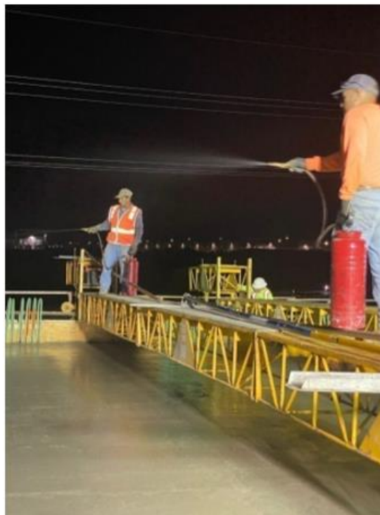
Figure 2.66: Applying Finishing Aid to the Concrete Surface
