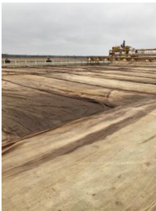
Figure 2.48: Burlap Placement on the Deck
