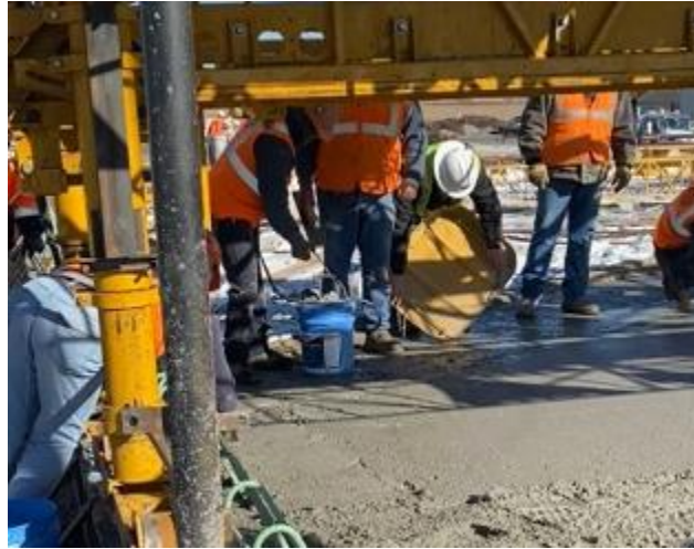
Figure 2.58: Applying Finishing Aid to the Concrete Surface
