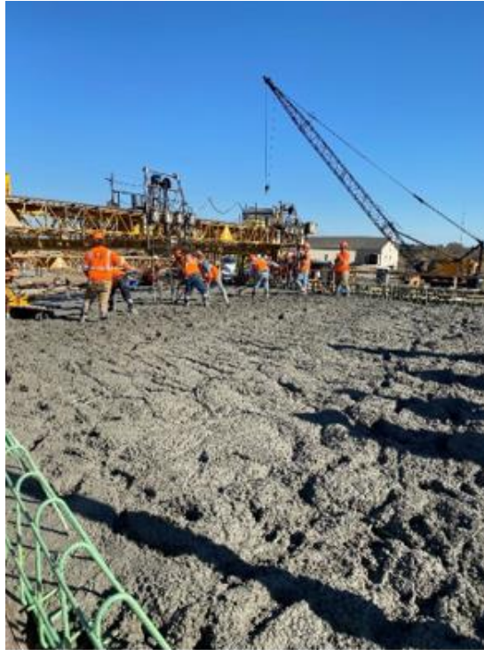
Figure 2.52: Concrete Left Unconsolidated and Unprotected Due to Inoperable Roller Screed
