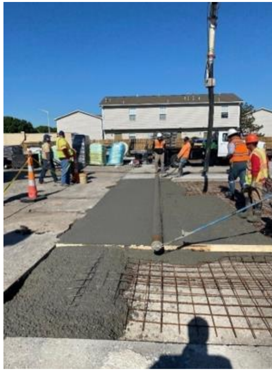
Figure 2.63: The Qualification Slab Placement Equipment
