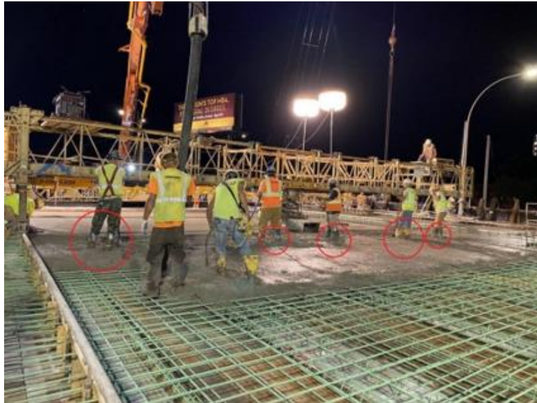
Figure 2.23: Walking Observed on Freshly Consolidated Concrete
