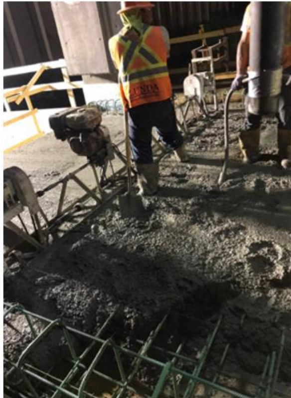
Figure 2.10: Placement, Consolidation, and Finishing of MN-IC-LC-HPC-5
