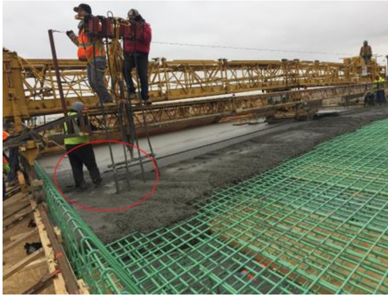
Figure 2.46: Walking Through Consolidated Concrete
