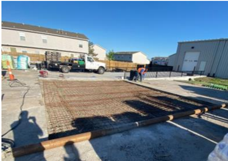
Figure 2.62: The Qualification Slab for KS-IC-LC-HPC-3
