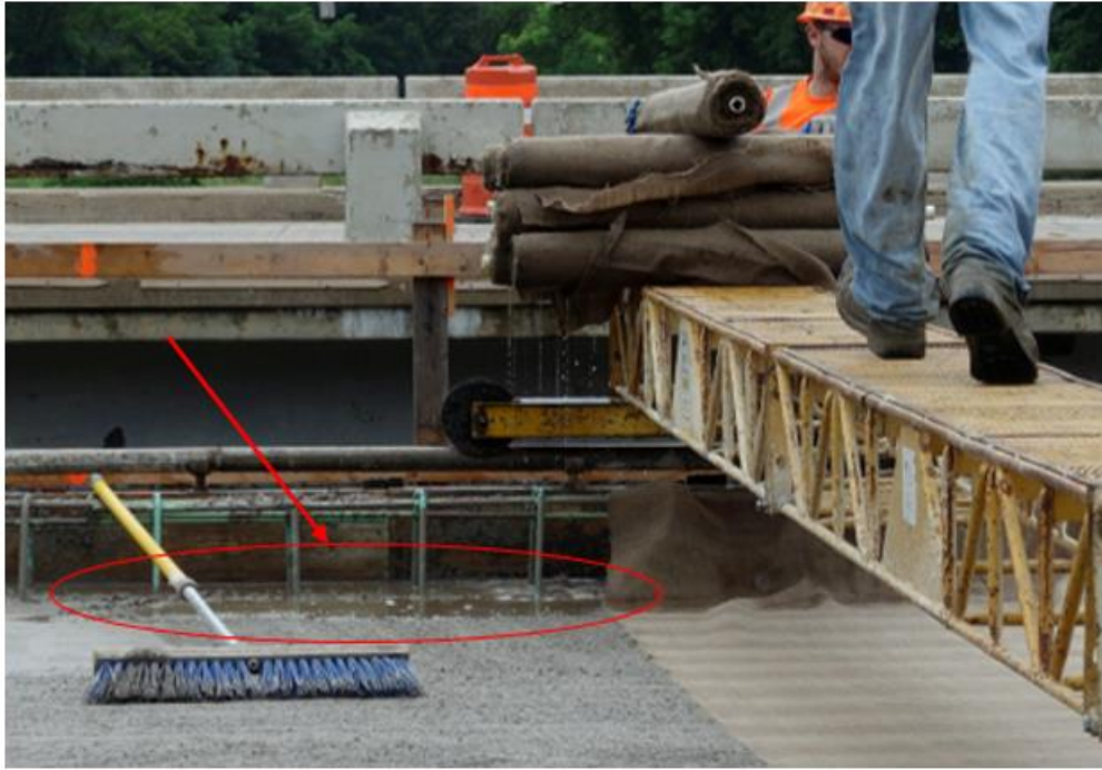
Figure 2.4: Water from Burlap Dripping onto the Deck
