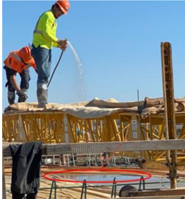
Figure 2.55: Ponding Observed on the Deck
