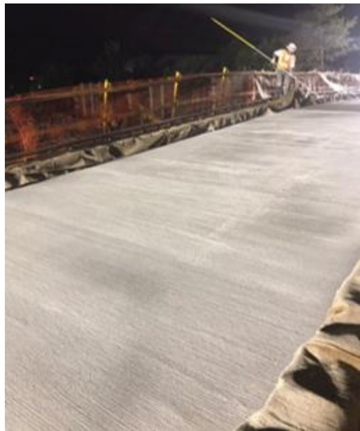
Figure 2.15: Burlap Placement on the Barrier Reinforcement
