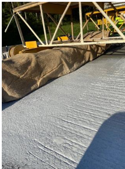
Figure 2.38: Burlap Placement on the Barrier Reinforcement
