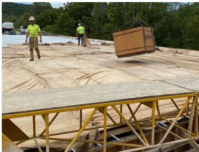
Figure 2.40: Wet Curing Application on MN-IC-LC-HPC-9
