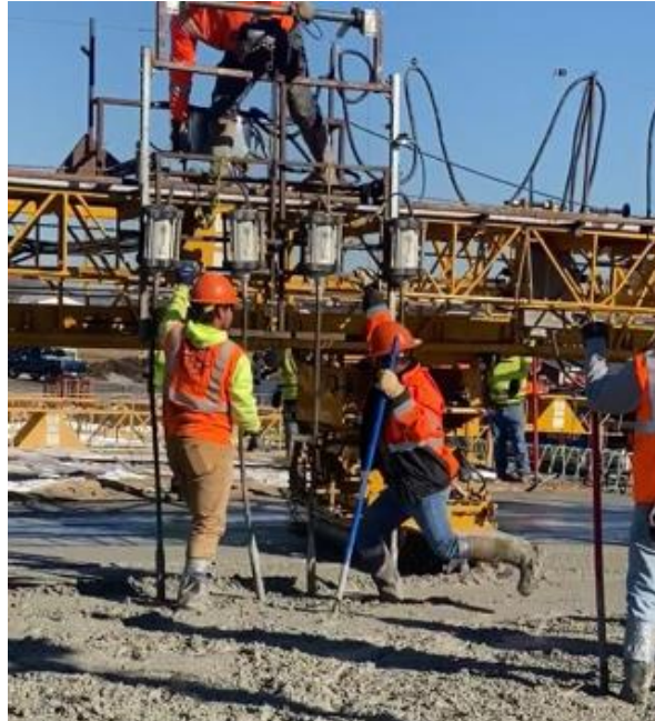
Figure 2.57: Malfunctioning of the Machine-Mounted Gang Vibrators
