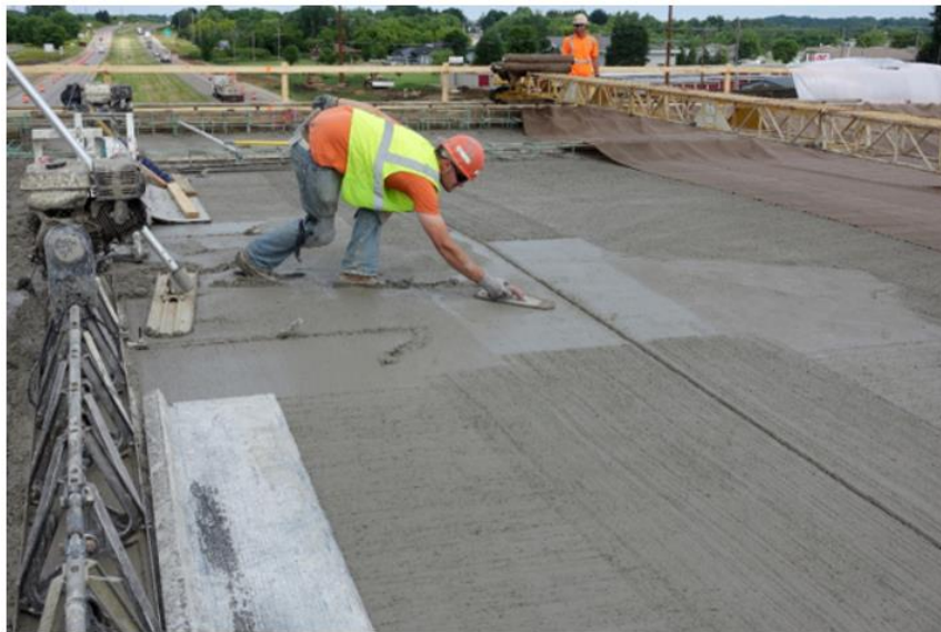
Figure 2.5: Walking through Freshly Consolidated Concrete
