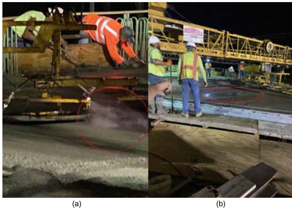
Figure 2.64: Excessive Water on the Deck (a) Unadjusted Nozzles; (b) Ponded Water on the Surface
