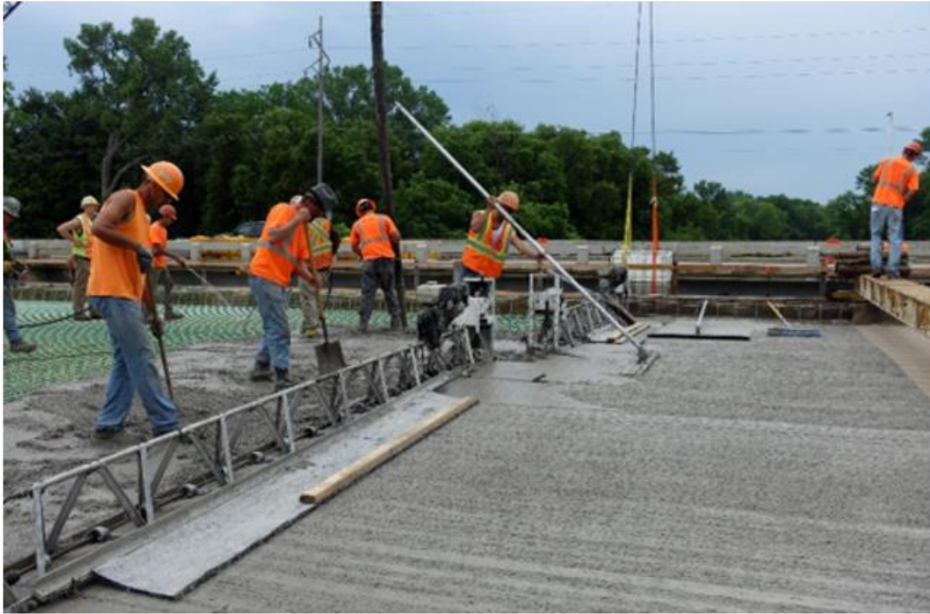
Figure 2.3: Finishing Equipment for MN-IC-LC-HPC-2 Subdeck
