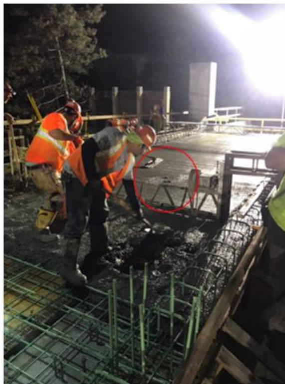
Figure 2.11: Holes in the Concrete Surface Duo to Rapid Removal of the Spud Vibrator
