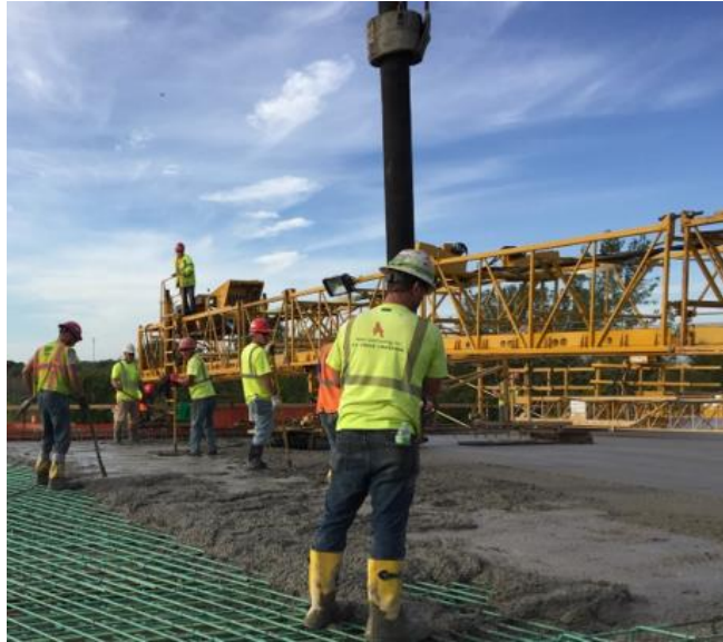
Figure 2.17: Placing, Consolidation, and Finishing Equipment
