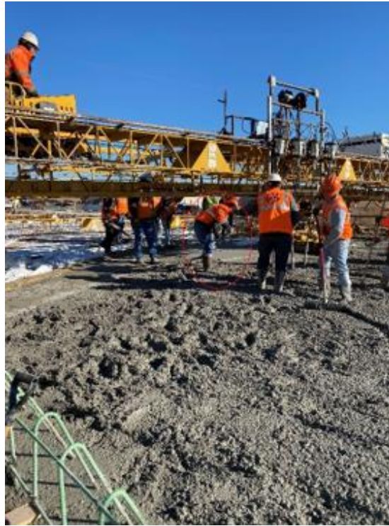
Figure 2.56: Walking Observed on Freshly Consolidated Concrete
