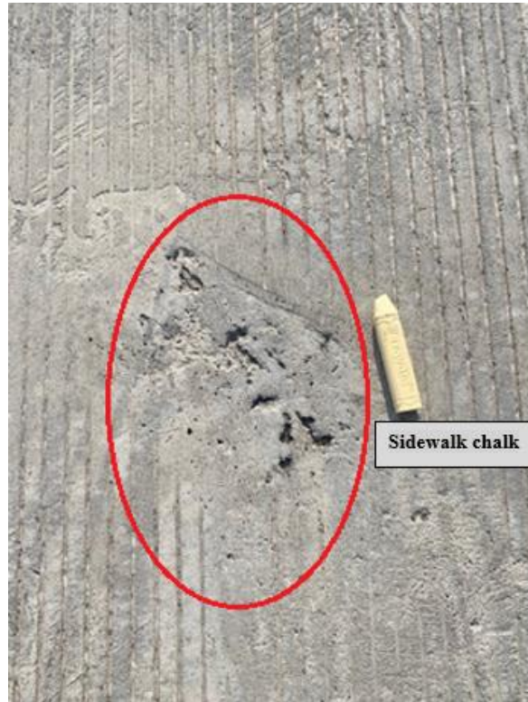
Figure 3.34: Surface Damage Observed on KS-IC-LC-HPC-2-P1
