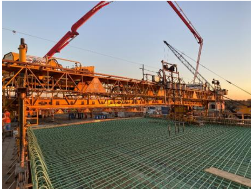
Figure 2.50: Consolidation and Finishing Equipment
