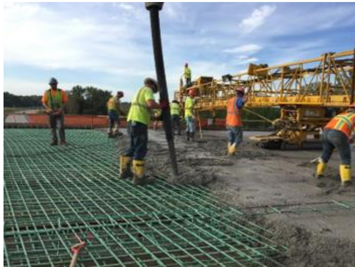
Figure 2.18: Walking Through Consolidated Concrete
