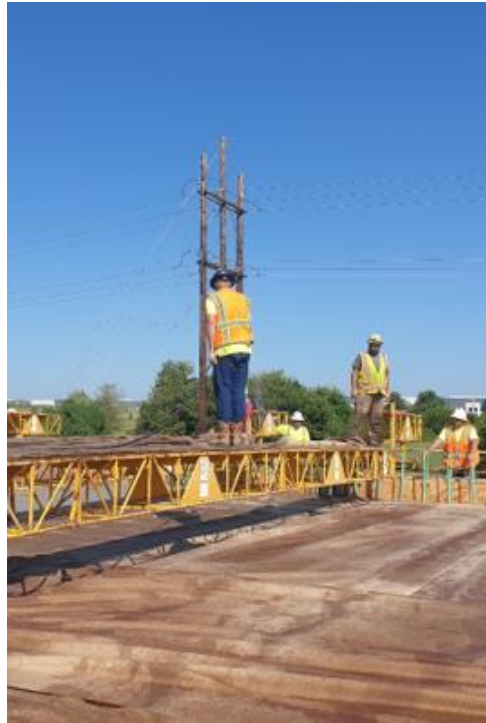
Figure 2.68: Rewetting the Burlap on the Deck
