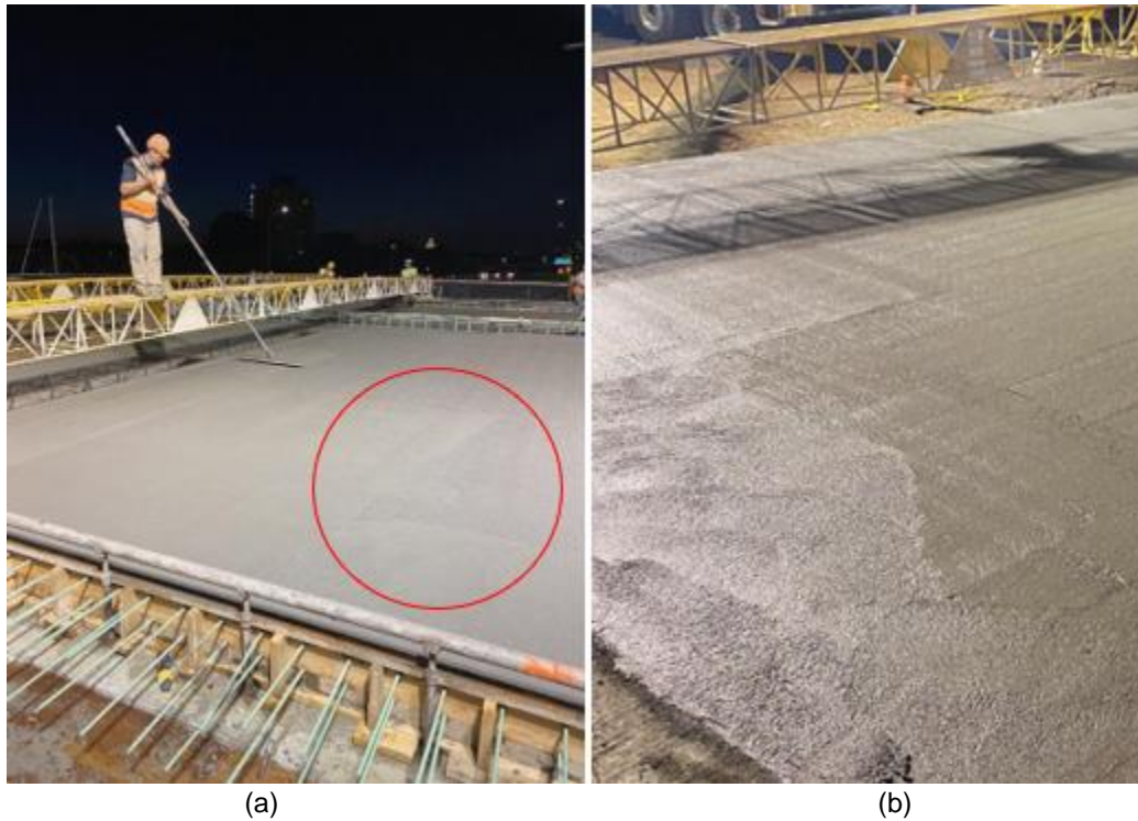
Figure 2.24: Bull Floating the Deck in the Presence of Bleed Water (a) An Overview; (b) A Close-Up View
