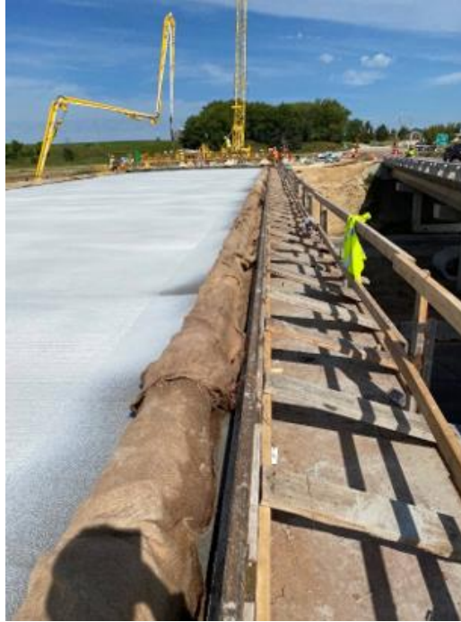
Figure 2.33: Burlap Placement on the Barrier Reinforcement
