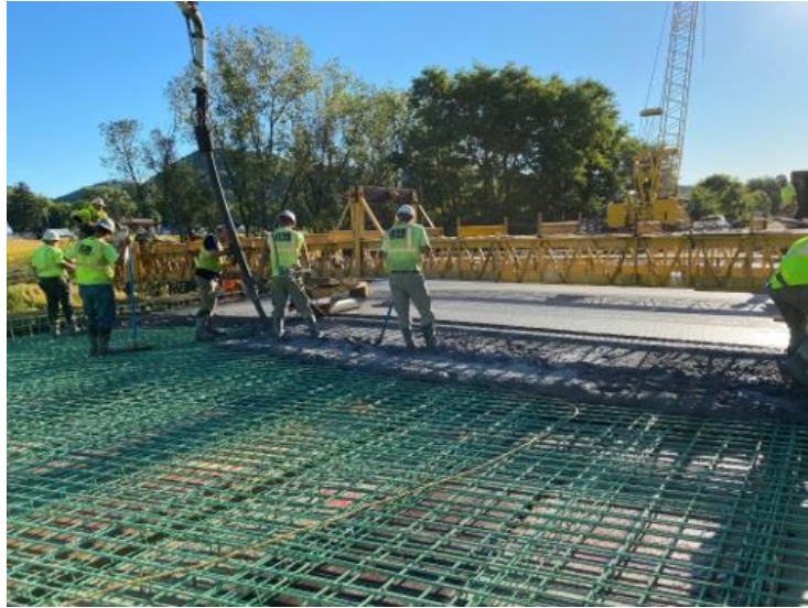
Figure 2.36: MN-IC-LC-HPC-9 Placement
