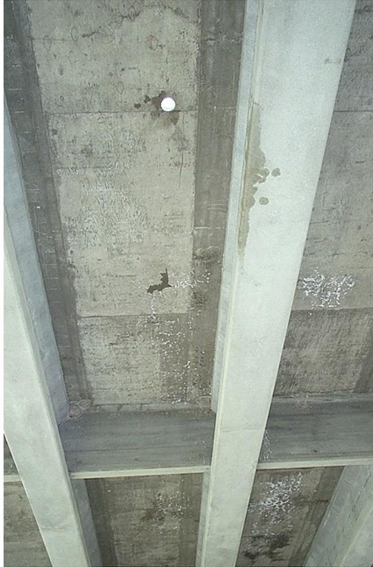
**Figure 4.28. Photograph from beneath bridge deck after coring operation. Hole from core T-2 is visible. Dampness permeating through cracks visible beneath the area of core T-1. White efflorescence common in areas directly below regions covered with cold patch material.**
