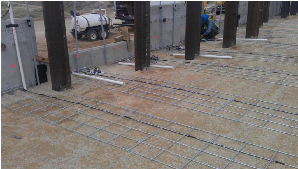
**Figure 4.6 Instrumented grids being placed in the fill.**
