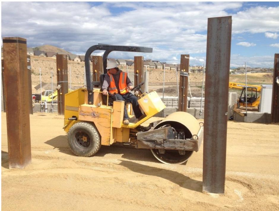
**Figure 3.9: Roller compaction between test and reaction piles.**
