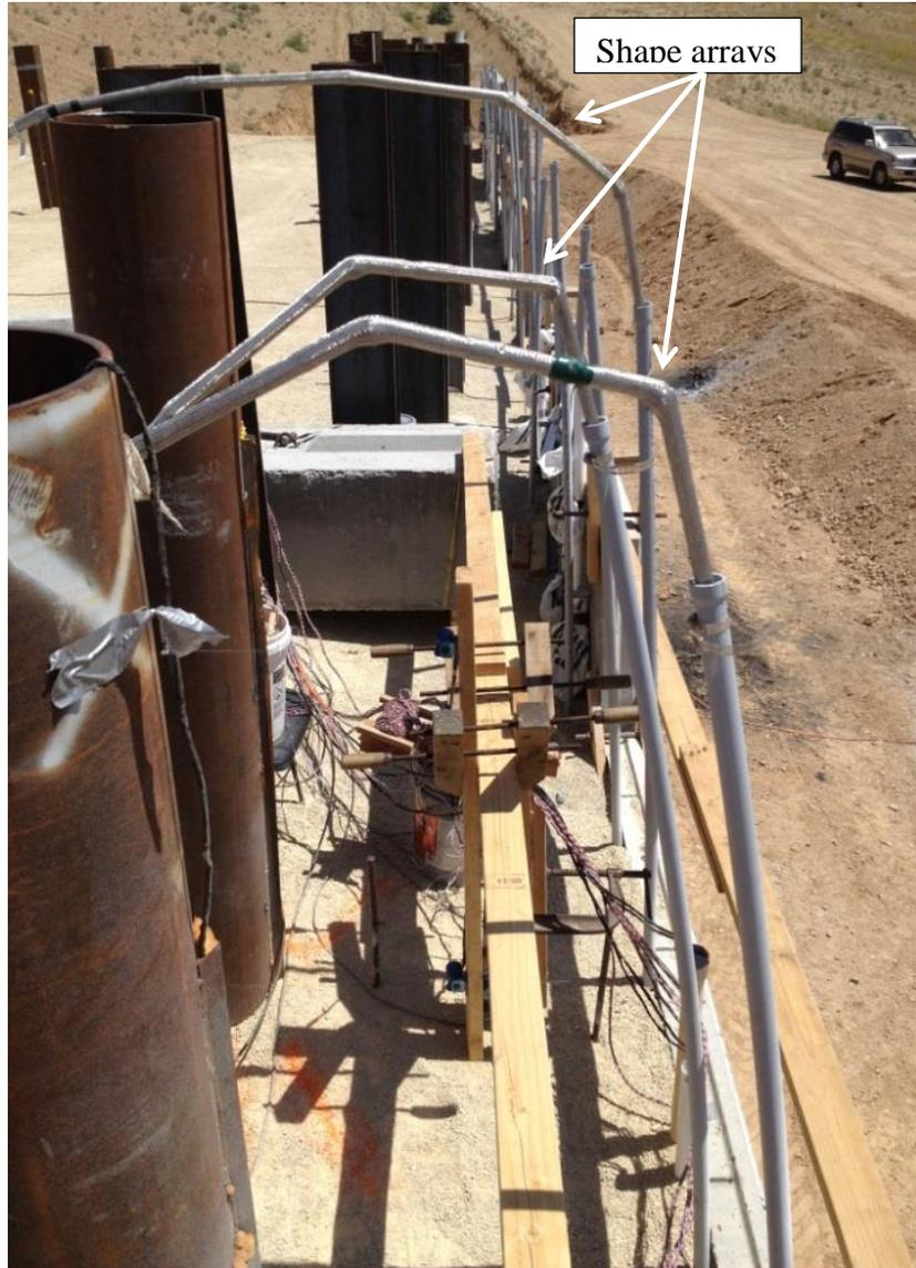
**Figure 4.12: Photograph of shape arrays in place behind the face of the wall.**
