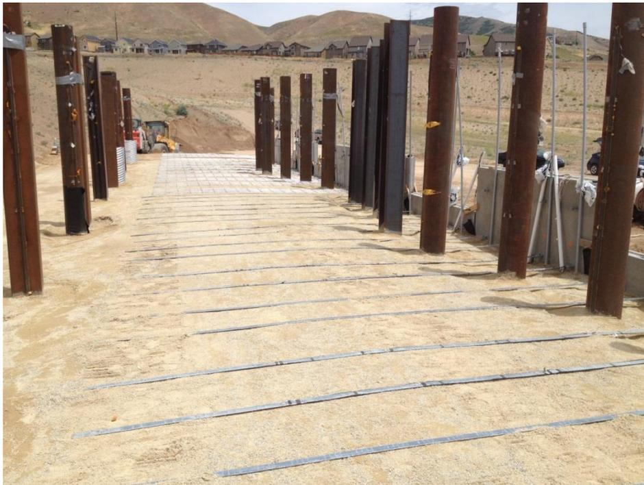
**Figure 3.6: Ribbed strip reinforcements and welded wire grid reinforcements.**
