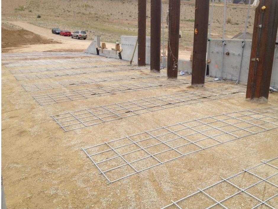
**Figure 3.7: Welded wire grid reinforcements.**
