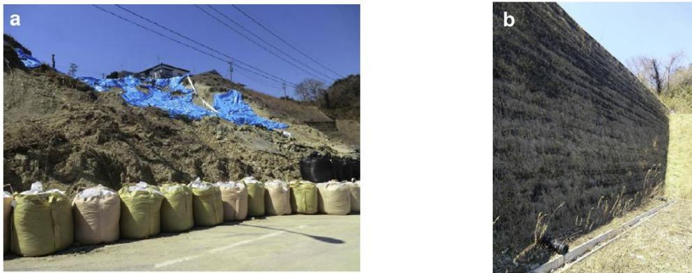
**Figure 2.5: (a) Collapse of unreinforced embankment and (b) undamaged GRS RW at Yamamoto town, Miyagi (Koseki 2012).**
