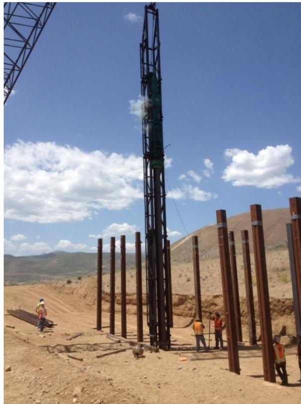
**Figure 3.14: Pile driving using a diesel hammer.**
