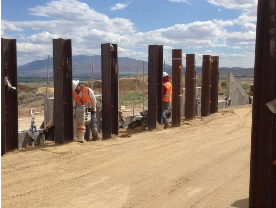
**Figure 3.10: Jumping jacks for compaction around test piles and vibratory plate for compaction within 3 ft. of wall.**
