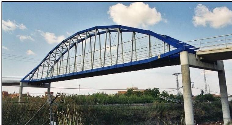
**Figure 5: Glass FRP arched pedestrian bridge, Lleida, Spain (Fiberline Composites, 2019).**
