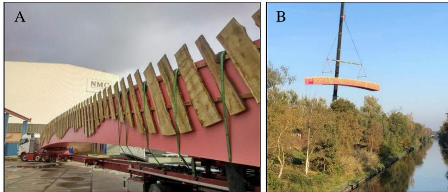
**Figure 10: A) FRP uni-mold bridge is delivered in one piece from the factory to the construction site; B) bridge is installed using one crane (FiberCore Europe, 2019b).**
