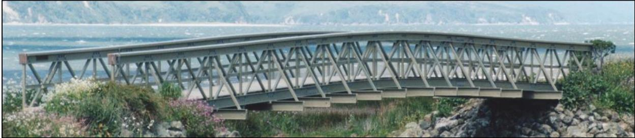
**Figure 4: Pultrusion-style pedestrian bridge in Marshall, CA. (Creative Pultrusions Inc., 2019).**
