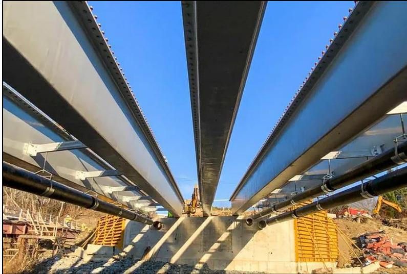
**Figure 36: The CT girder bridge system installed during first construction in Hampden, Maine, 2020 (Advanced Infrastructure Technologies, 2020).**
