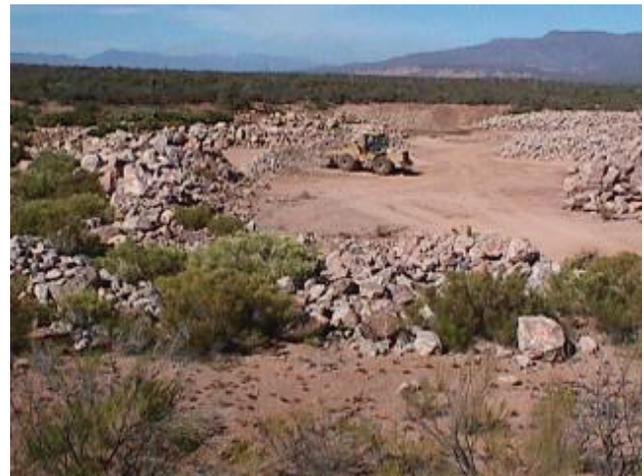
**FIGURE 36. CONTRACTOR SORTING MATERIAL FOR RIP RAP AND AGGREGATE PRODUCTION IN ARIZONA, STATE ROUTE 188, AND ON THE TONTO NATIONAL FOREST. PHOTO CREDIT: T. BRENNAN.**
