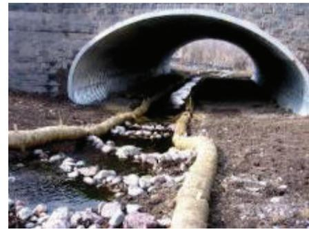
**FIGURE 30. THIS CULVERT ON US 93 NORTH WAS ENLARGED TO ACCOMMODATE WILDLIFE PASSAGE IN ADDITION TO WATER FLOW.**
