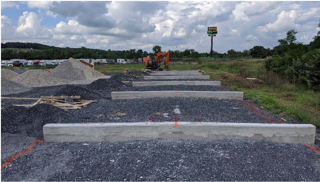
Figure 3. Installed section dividers
