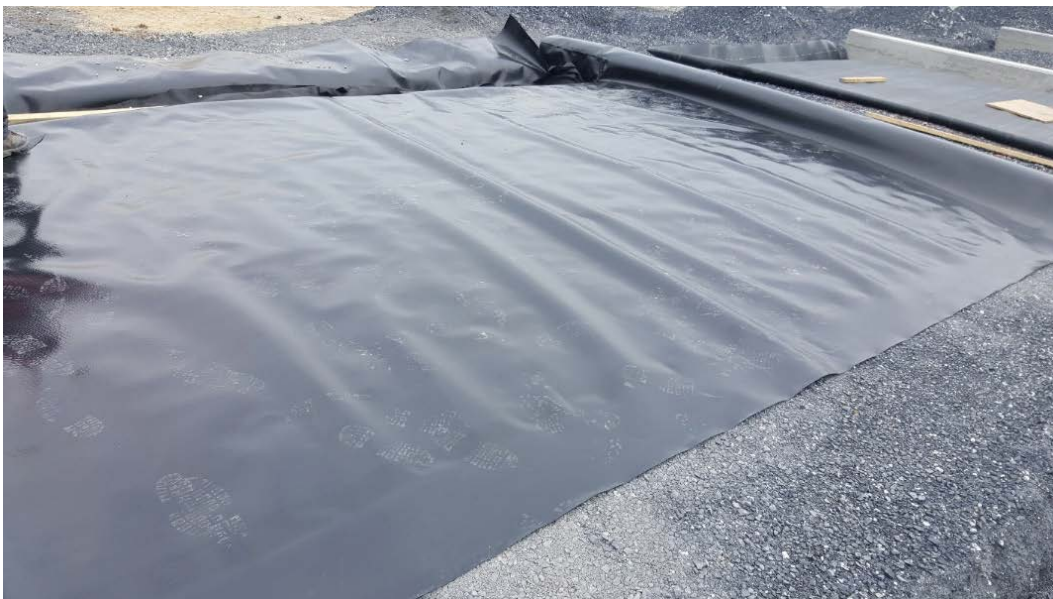
Figure 4. Installation of the 40 mil HDPE geomembrane liner
