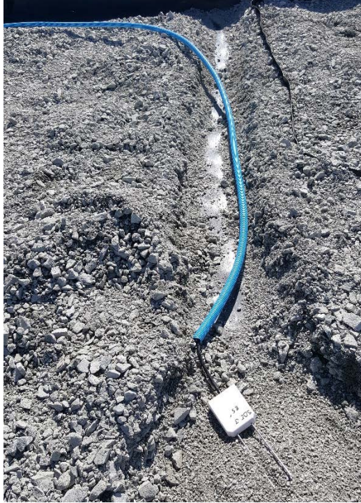
Figure 9. Installation of volumetric moisture content sensor within the base course
