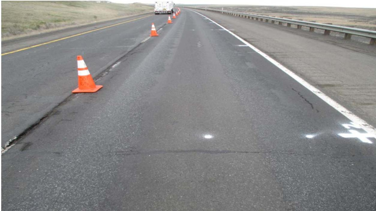
**Figure 12. Image of station 200 prior to coring in 2019. The white dot paint marks are locations for FWD measurements.**
