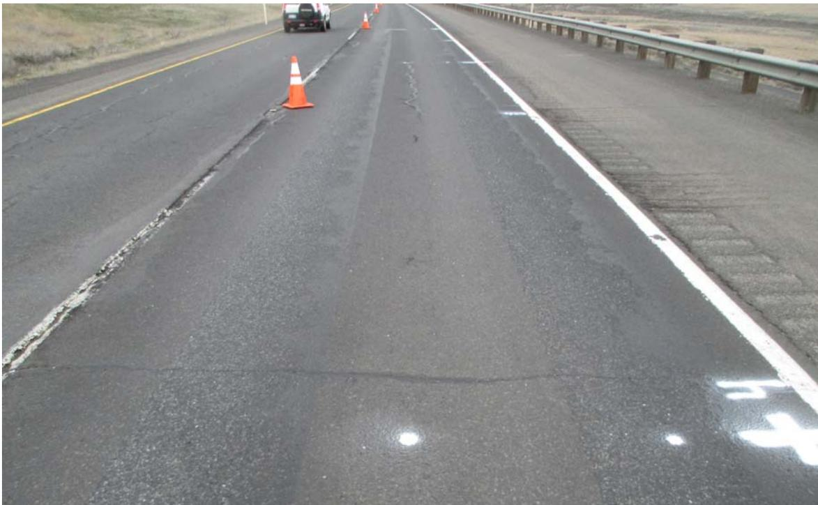
**Figure 18. Condition of the pavement at station 400 prior to coring. The white dots are FWD test locations.**
