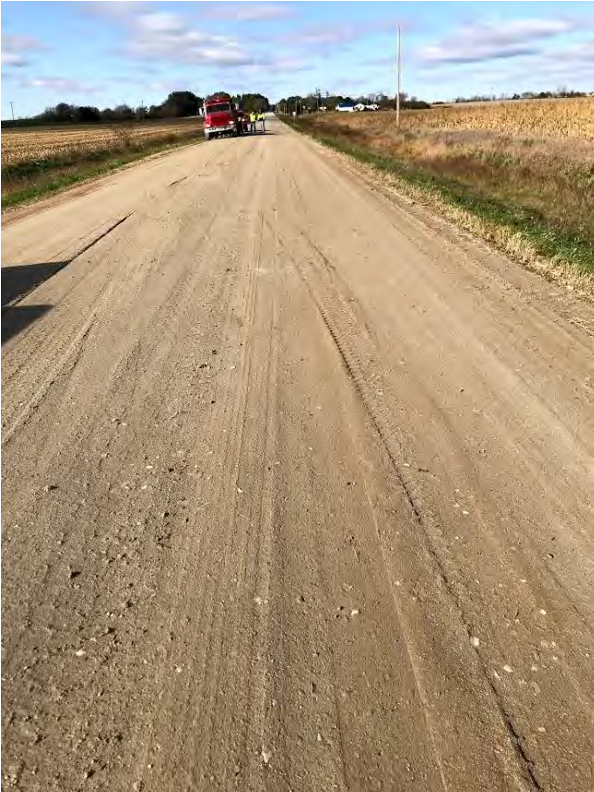
Appendix A – Figure 10. Moscow section in Boone County after construction, November 2019
