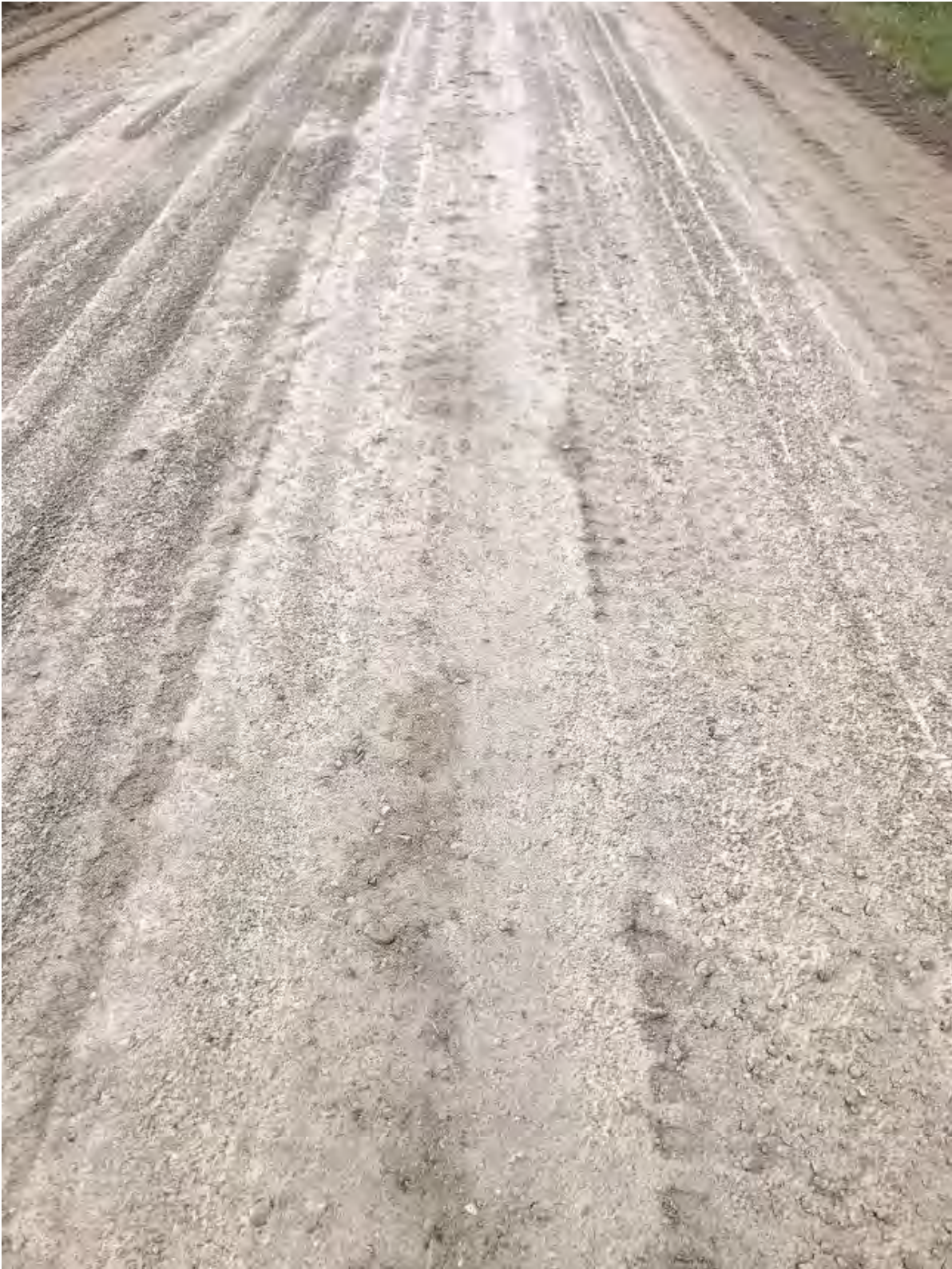
Appendix A – Figure 18. Crescent section in Boone County after construction, November 2019
