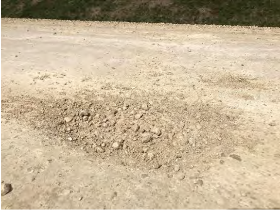
Figure 32. Distress types happened to the surface materials, (a) big pothole in middle of Moscow section in Jones County, (b) sever rutting in Moscow section in Jones County
