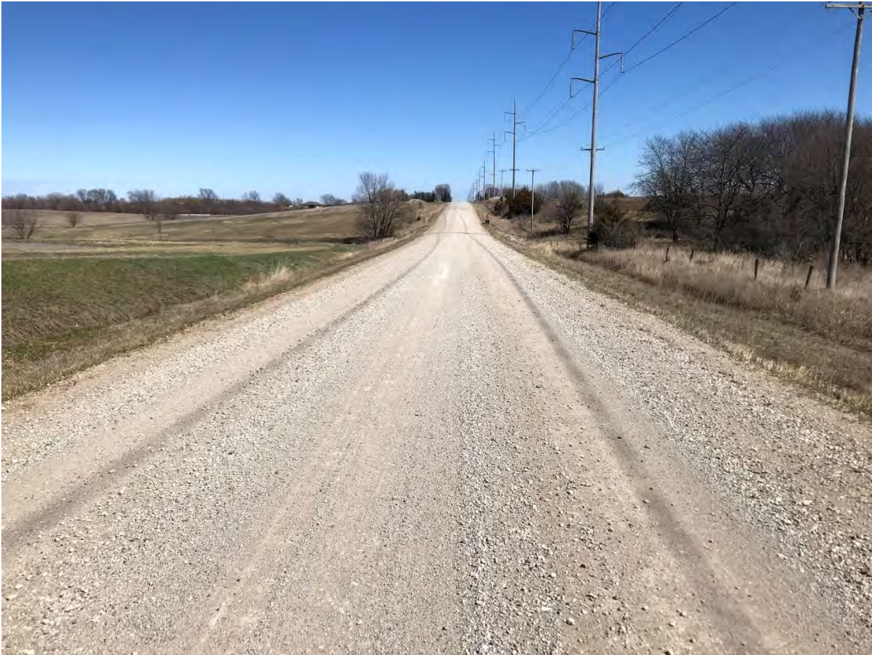
Appendix A – Figure 22. Control section in Boone County, March 2020
