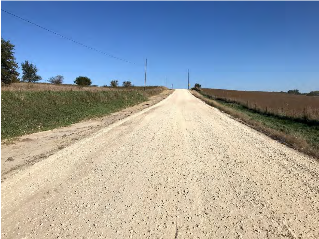
Appendix A – Figure 34. Control section in Jones County, November 2019
