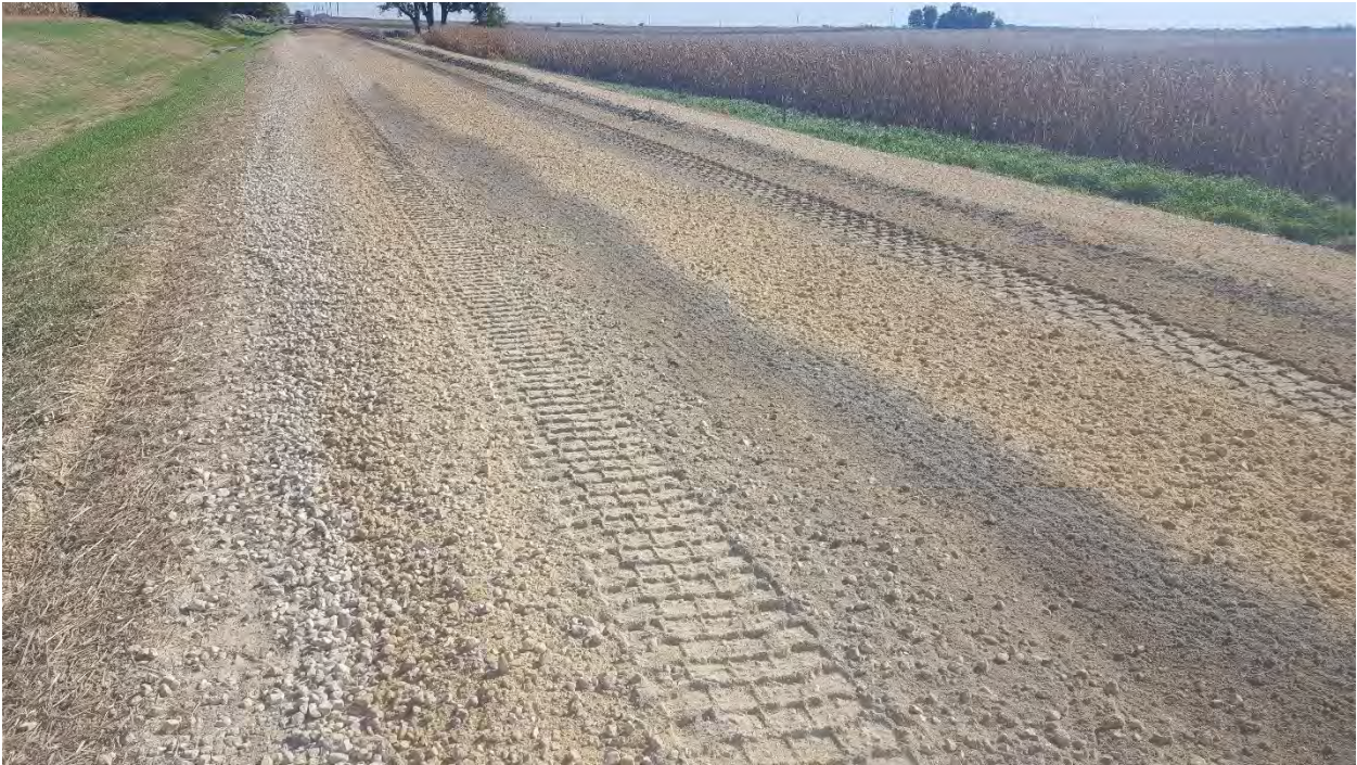
Appendix A – Figure 25. Moscow section in Jones County after construction, November 2019
