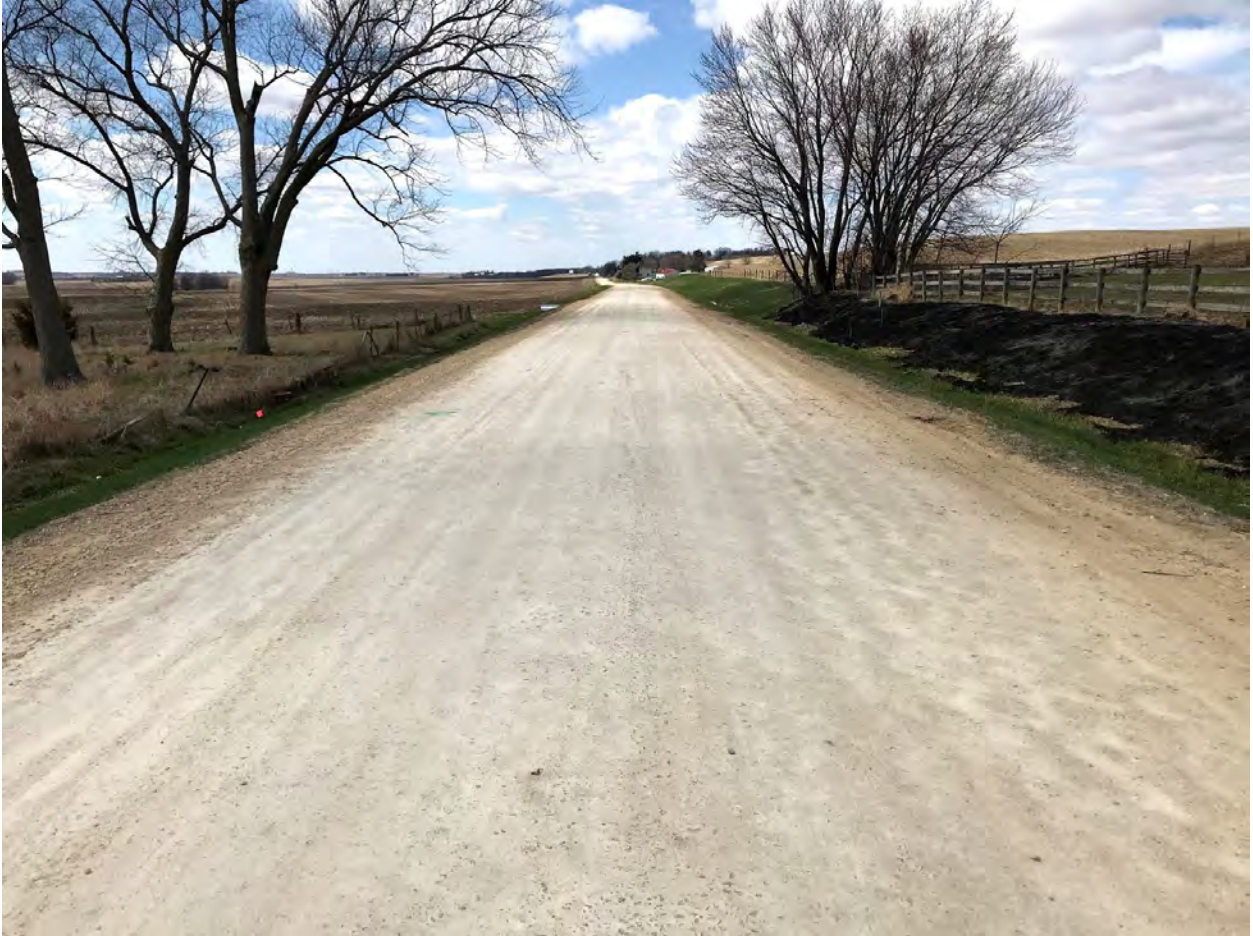
Appendix A – Figure 29. Clay Slurry section in Jones County, March 2020
