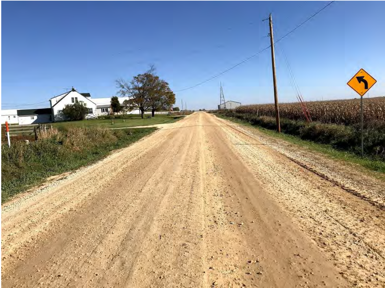
Appendix A – Figure 31. Limestone section in Jones County after construction, November 2019
