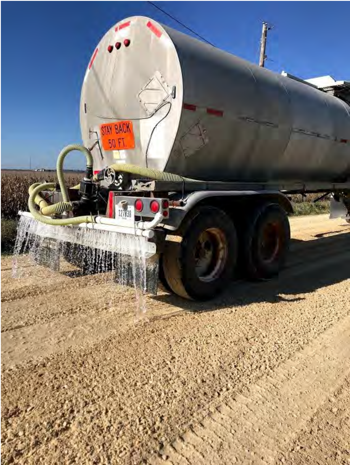
Appendix A – Figure 2. Water tank in Jones County
