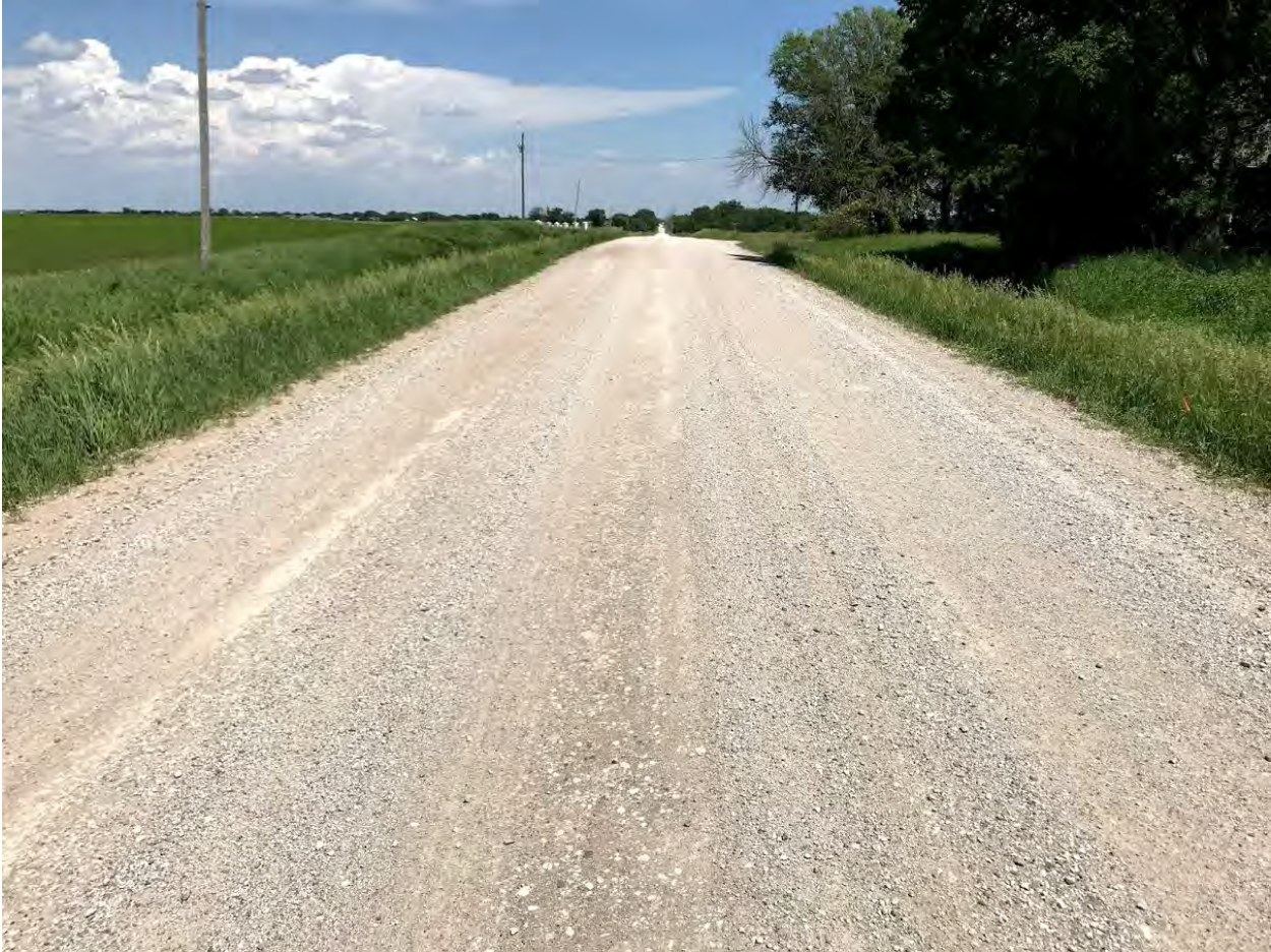
Appendix A – Figure 13. Moscow section in Boone County, June 2020
