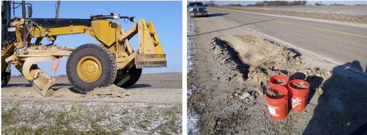
Figure 26: Motor Grader and Soil Sampling from CR G37 Located in Washington Co, IA
