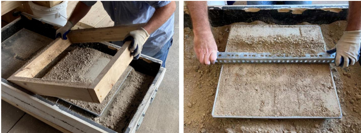
Figure 37: Preparation and Screeding of Compacted Soil Form
