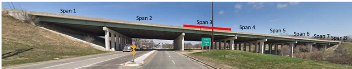
Figure . I-70 highway bridge (Eastbound)
