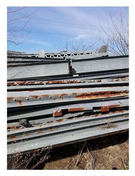
Figure 4 - Typical truss members obtained from INDOT with "real" pack-out and section loss
