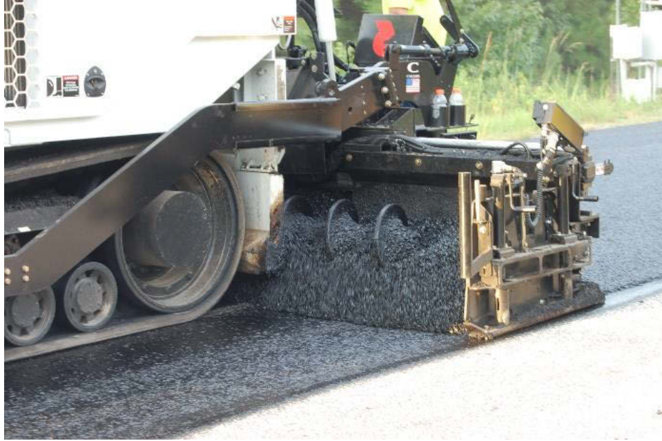
Figure 4 OGFC Placement in Section N9
