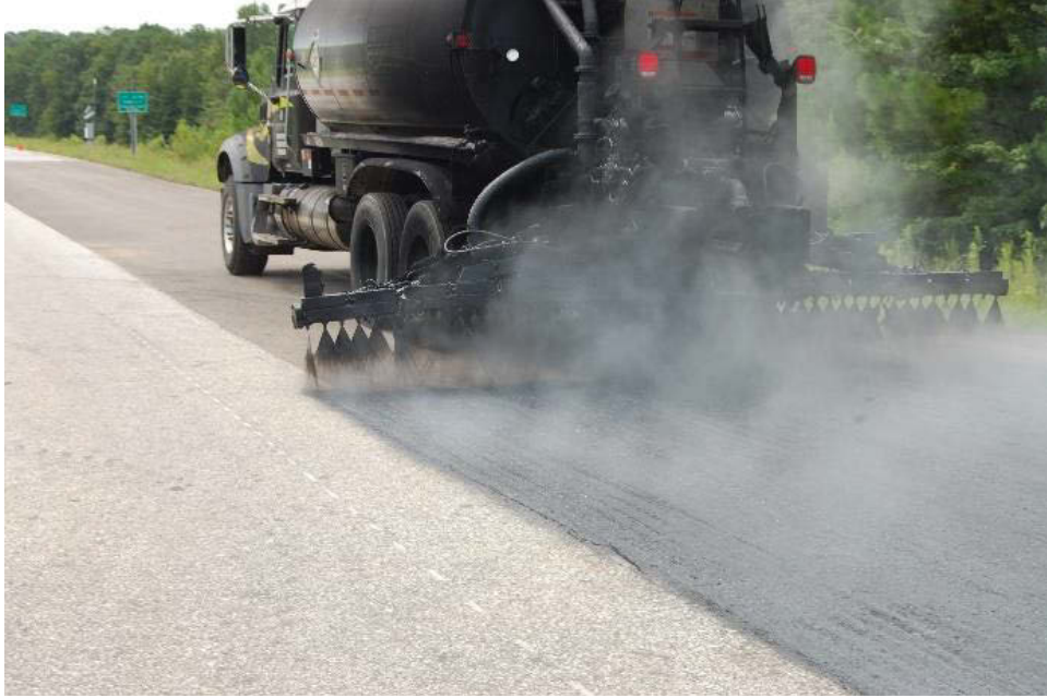
Figure 2 Application of Tack Coat on Section N9
