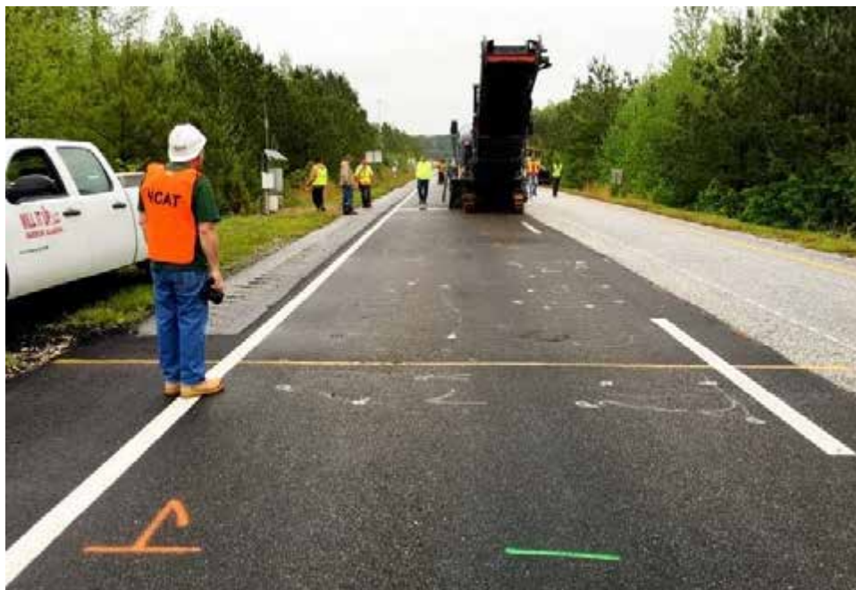
Figure 1 Milling of the Original Surface of Section N7
