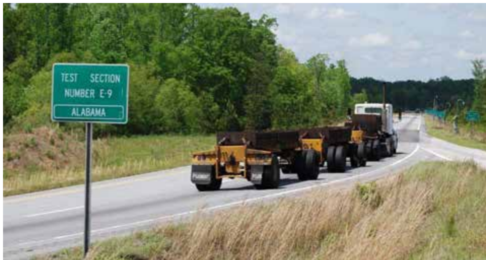
Figure 3 Heavily Loaded Triple-Trailer used for Accelerated Loading on the Test Track
