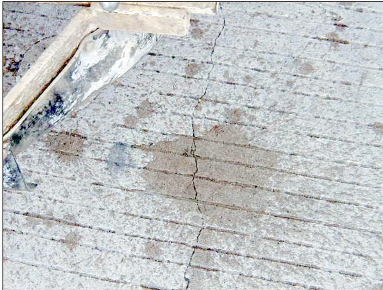
Figure IA-2: Photograph of crack in bridge deck.
