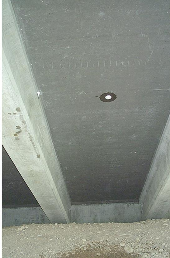
Figure S-3: Photograph from beneath bridge deck after coring operation, hole from core S-1 is clearly visible, light coming through hole from core S-2 is partly obscured by the pre-stressed beam.
