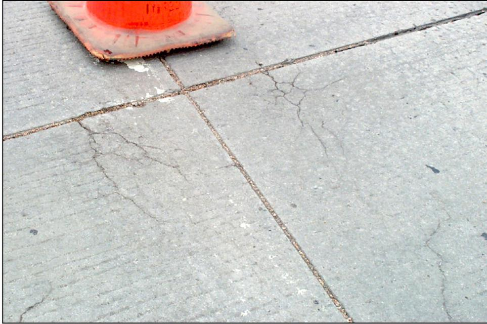
Figure CO-1: Photograph of cracks in pavement.
