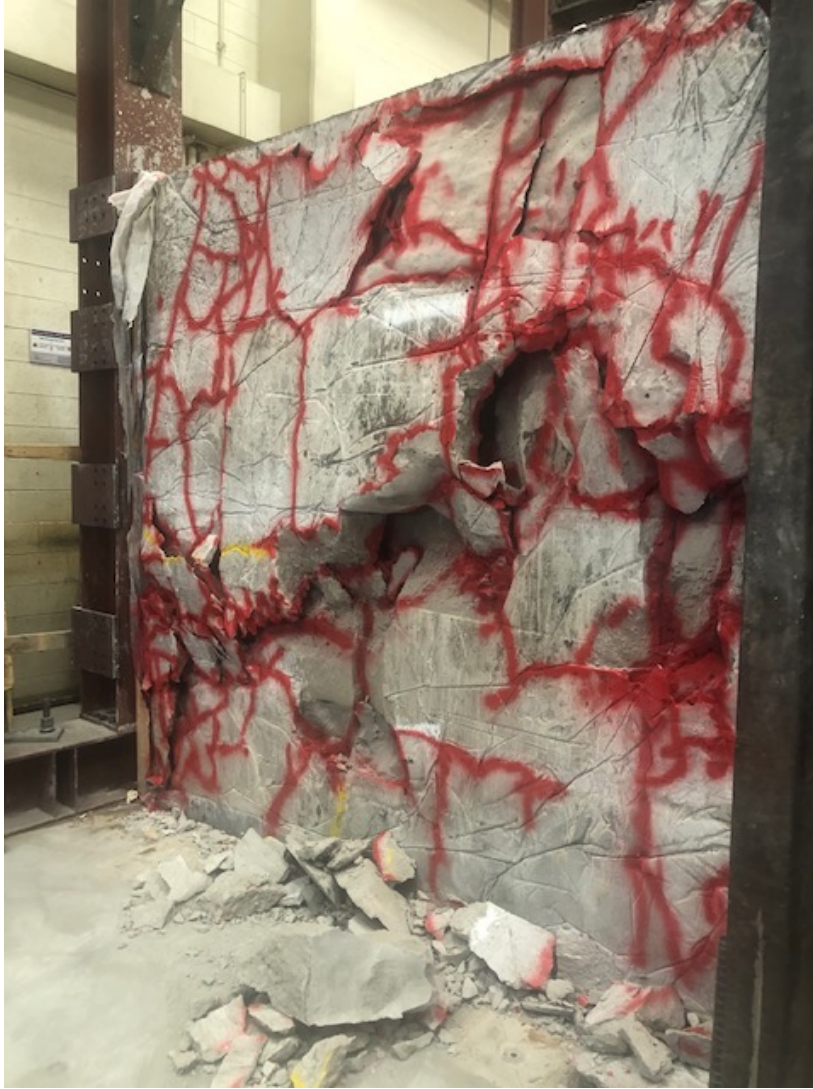
Fig. 13. Photograph of the crack pattern in the LCC on the free face opposite to the MSE retaining wall side.
