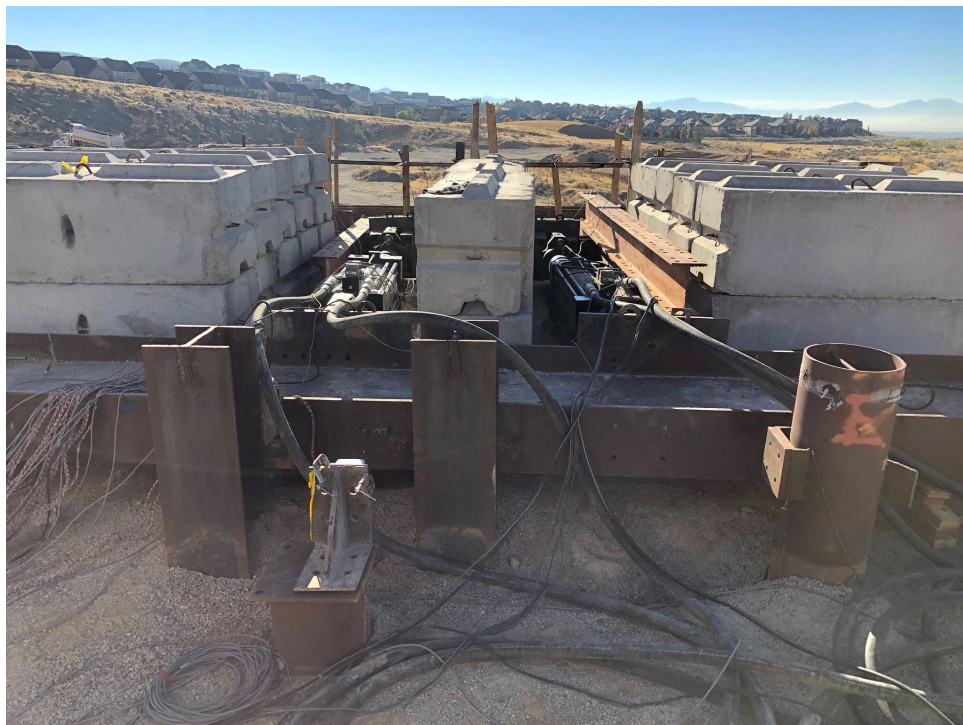
Fig. 2: Grouped test loading system.
