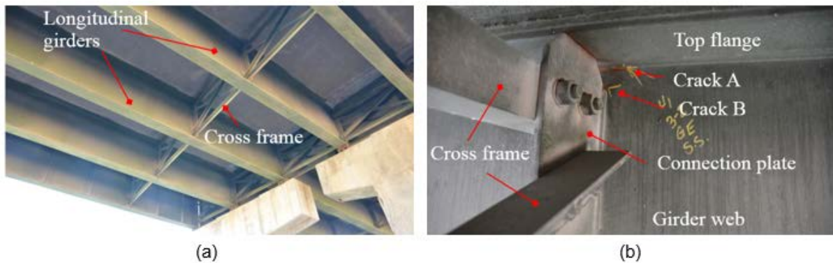
Figure 4.2: (a) A Typical Structural Layout of a Steel Girder Bridge in the Field; (b) Representative Distortion-Induced Fatigue Cracks at the Web-Gap Region
