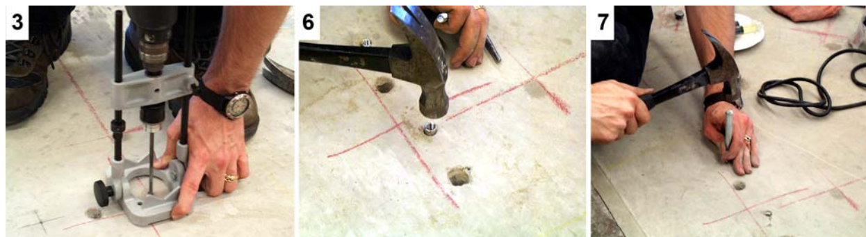
Figure 71. Photo. Concrete anchor installation, steps 3, 6, and 7.
