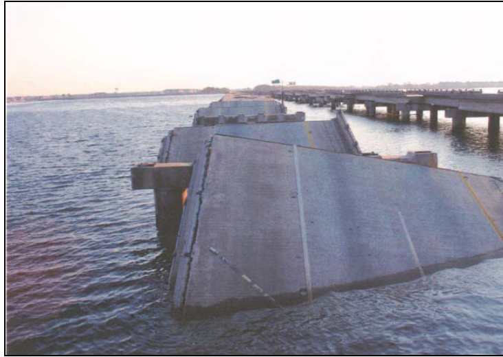
Figure 2.1 – I-10 Lake Ponchartrain Bridge after Hurricane Katrina Source: Volkert and Associates Damage Assessment
