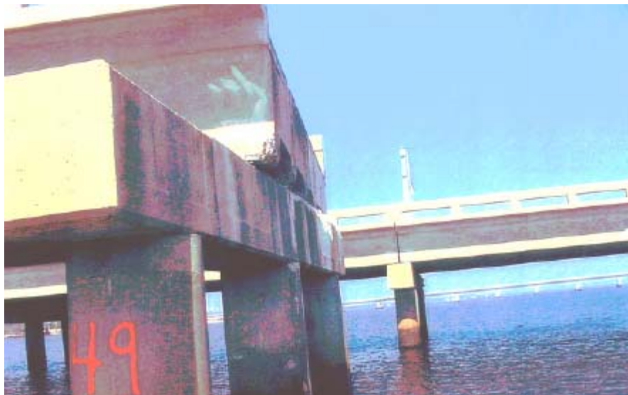
Span displaced laterally and longitudinally
