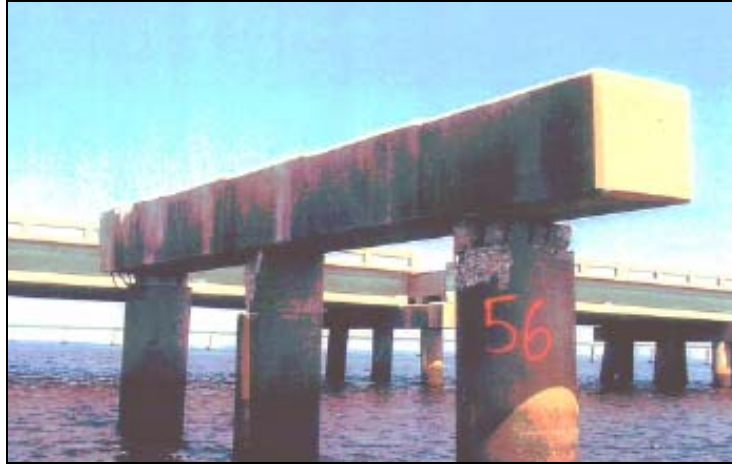
Figure 3.9 – Damage to a Pile to Bent Cap Connection on Escambia Bay Bridge Source: FDOT Damage Report
