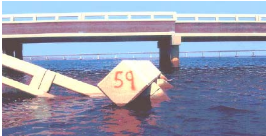
Bent failed longitudinally
