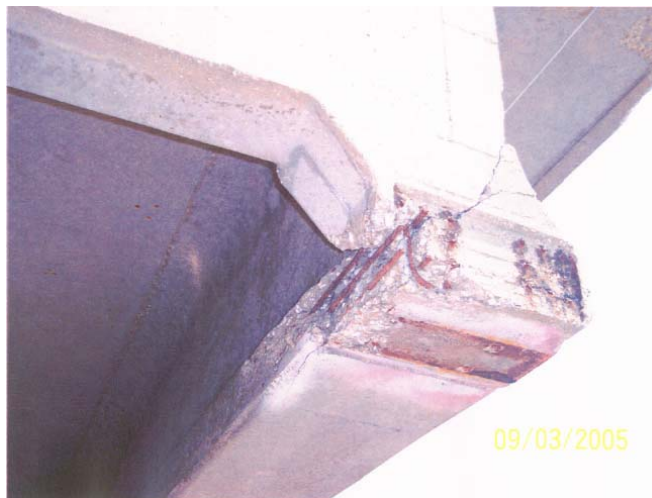
Fixed bearing at an exterior beam - (Bronze plate is still attached to pier, not shown) Straps holding the bronze plate to the beam failed while the anchor bolts remain intact
