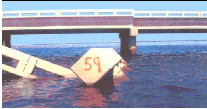
Figure 3.11 –Bent Exhibiting Longitudinal Damage on Escambia Bay Bridge Source: FDOT Damage Report
