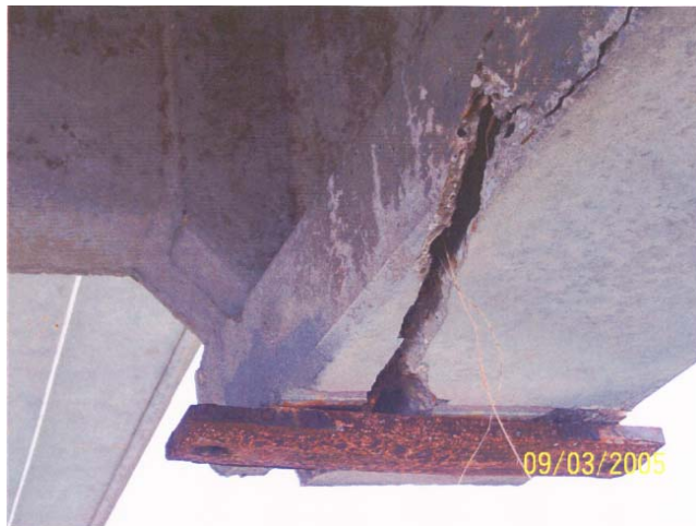
Fixed bearing at an exterior beam - Bronze plate is still attached to the beam Straps holding the bronze plate to the beam are intact while the anchor bolts failed
