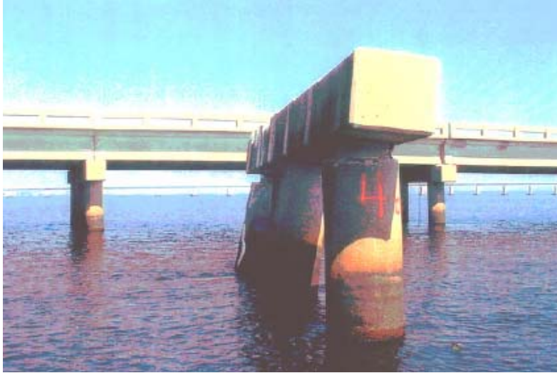
Bent deformed longitudinally
