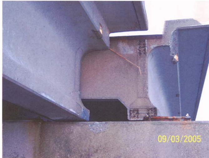
Fixed bearing at an exterior beam - Bronze plate still attached to pier Straps holding the bronze plate to the beam failed while the anchor bolts remain intact
