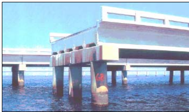
Figure 3.12 – Longitudinally Displaced Span on Escambia Bay Bridge Source: FDOT Damage Report
