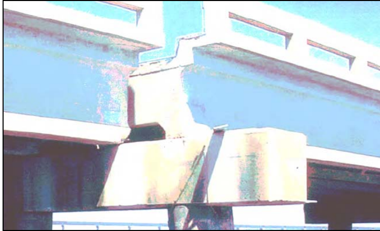
Figure 3.3 – Bent Cap with Bearing Plate Partially Attached on Escambia Bay Bridge Source: FDOT Damage Report
