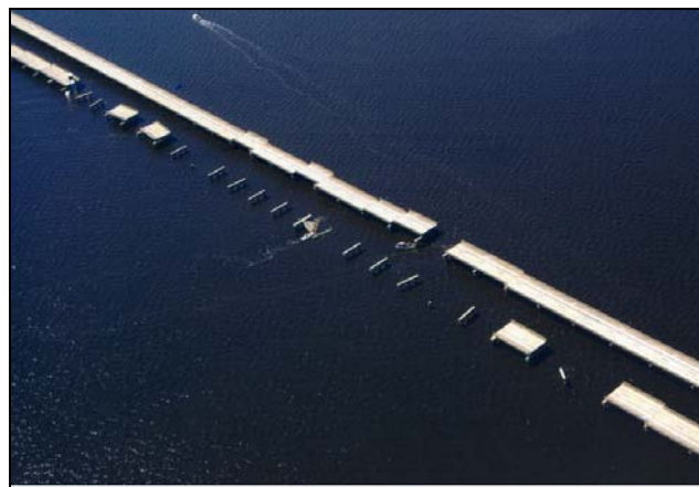
Figure 3.1 – I-10 Escambia Bay Bridge after Hurricane Ivan Source: FDOT
