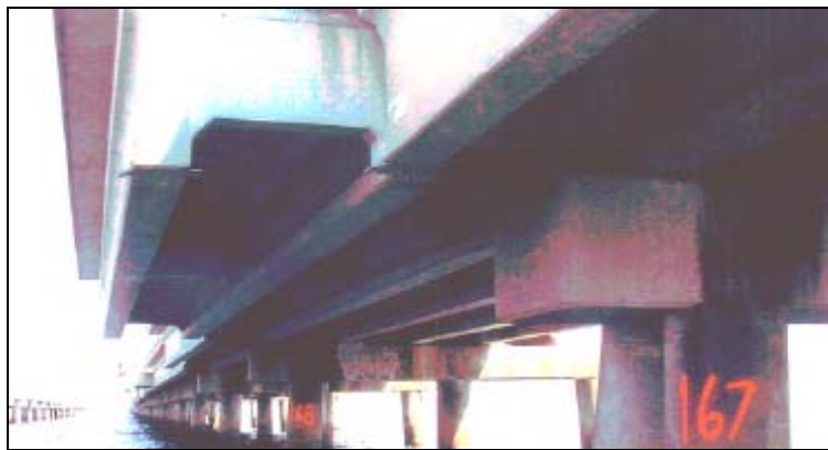
Figure 3.2 – Girders with Bearing Plates Intact on Escambia Bay Bridge Source: FDOT Damage Report
