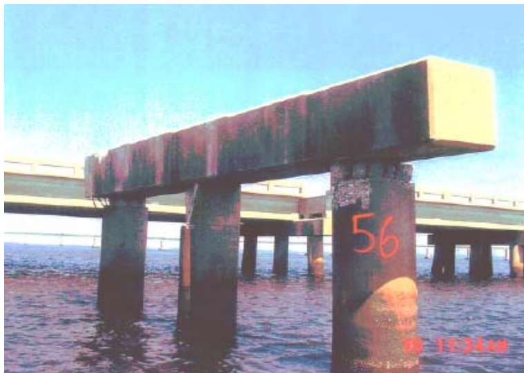
Bent with damaged pile to bent cap connection
