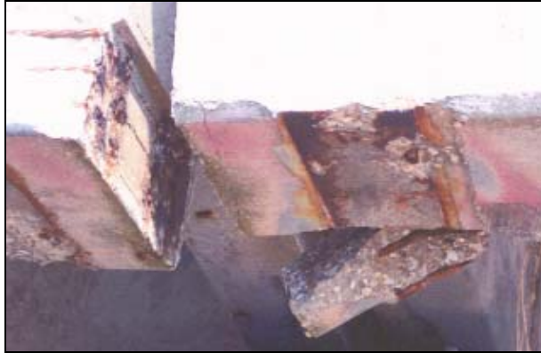
Figure 2.2 – Beams with Missing Bearing Plates on I-10 Lake Ponchartrain Bridge Source: Volkert and Associates Damage Assessment
