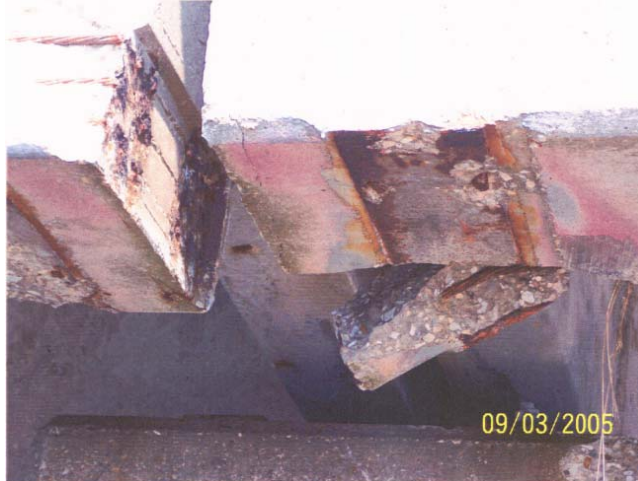
Fixed bearing at an exterior beam - (Bronze plate is still attached to pier, not shown) Straps holding the bronze plate to the beam failed while the anchor bolts remain intact
