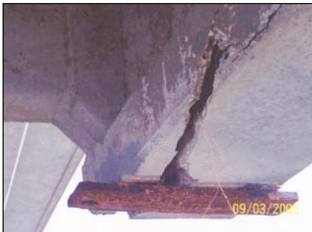
Figure 2.3 – Beam with Intact Bearing Plate on I-10 Lake Ponchartrain Bridge Source: Volkert and Associates Damage Assessment
