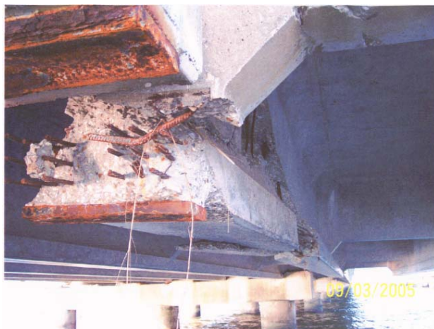
Free end any beam or fixed end interior beam (locations where plate not bolted to pier) Bronze plates remain attached to the beam through the straps (expected behavior)
