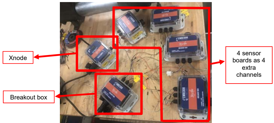
Figure 10. Connection of sensor boards to Xnode through breakout box
