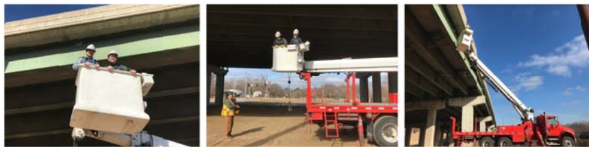
Figure 6. Field visit to the I-70 highway steel bridge.
